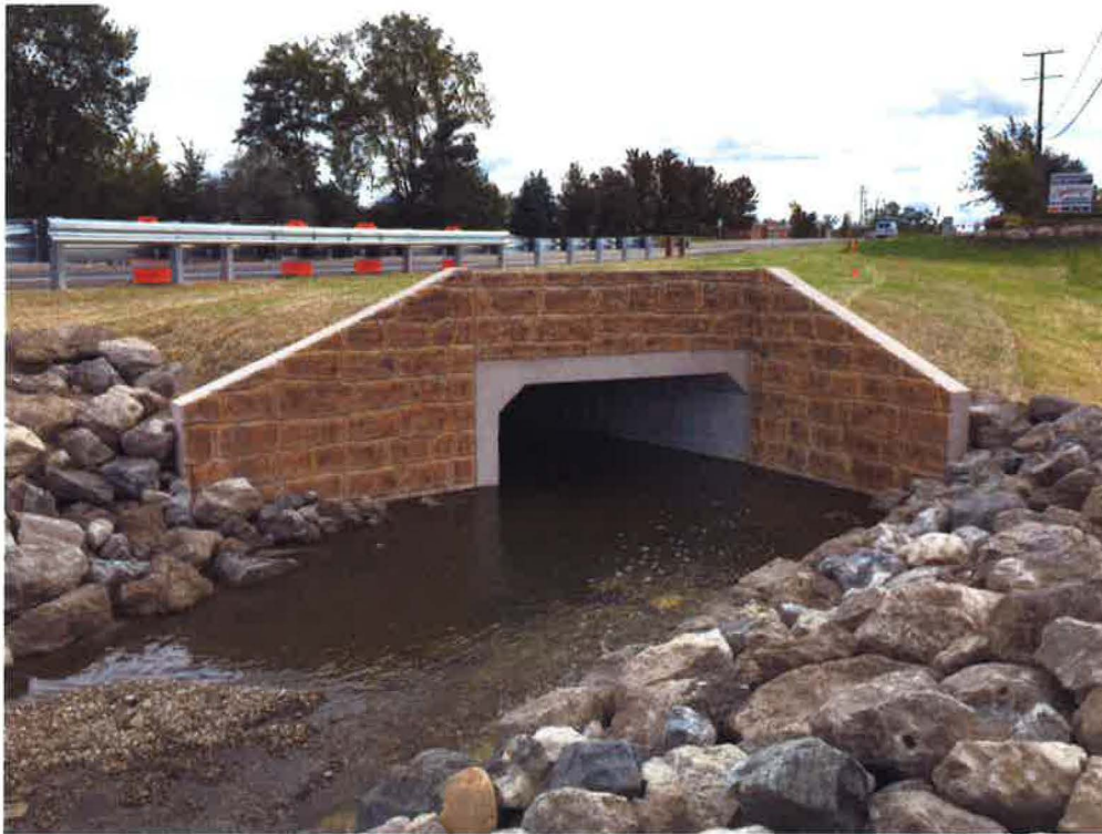
AFTER (West-Side, Inlet)
