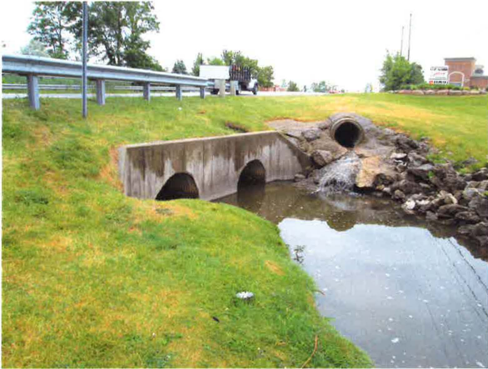
BEFORE (West-Side, Inlet)
