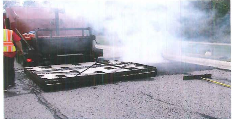
Heating and Reworking the Surface
