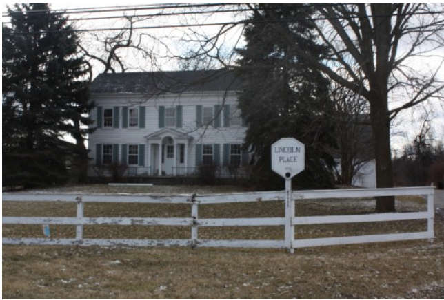
Lincoln Place, 47133 West Nine Mile (ca 1838)
