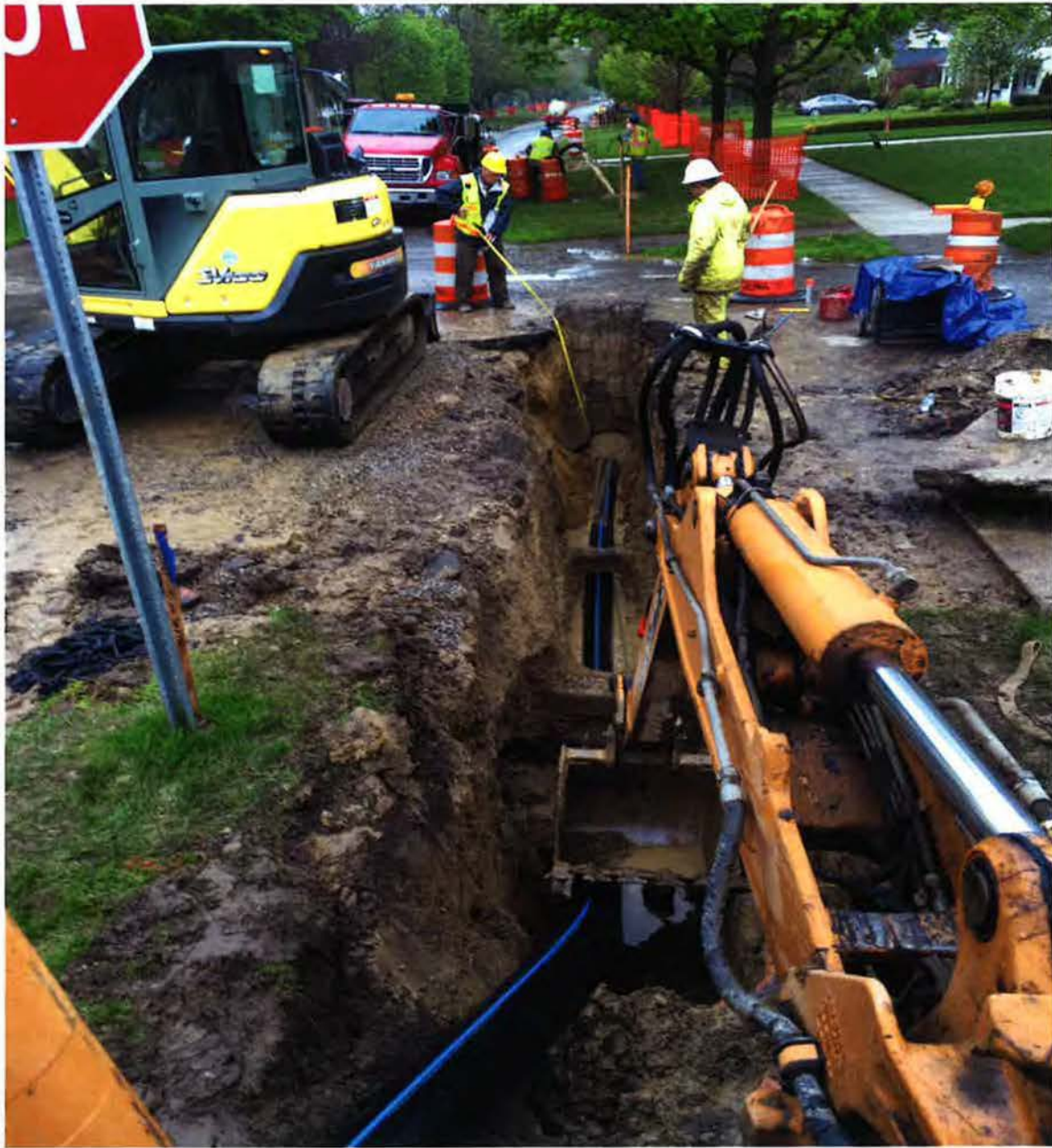
Tight utility crossing in Birmingham
