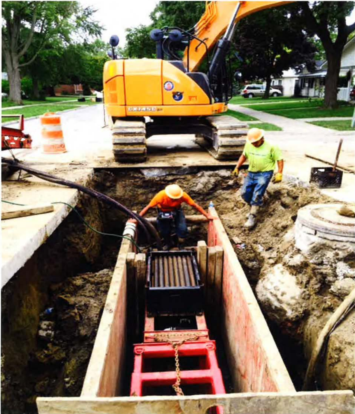
Typical Burst Pit Dearborn Heights
