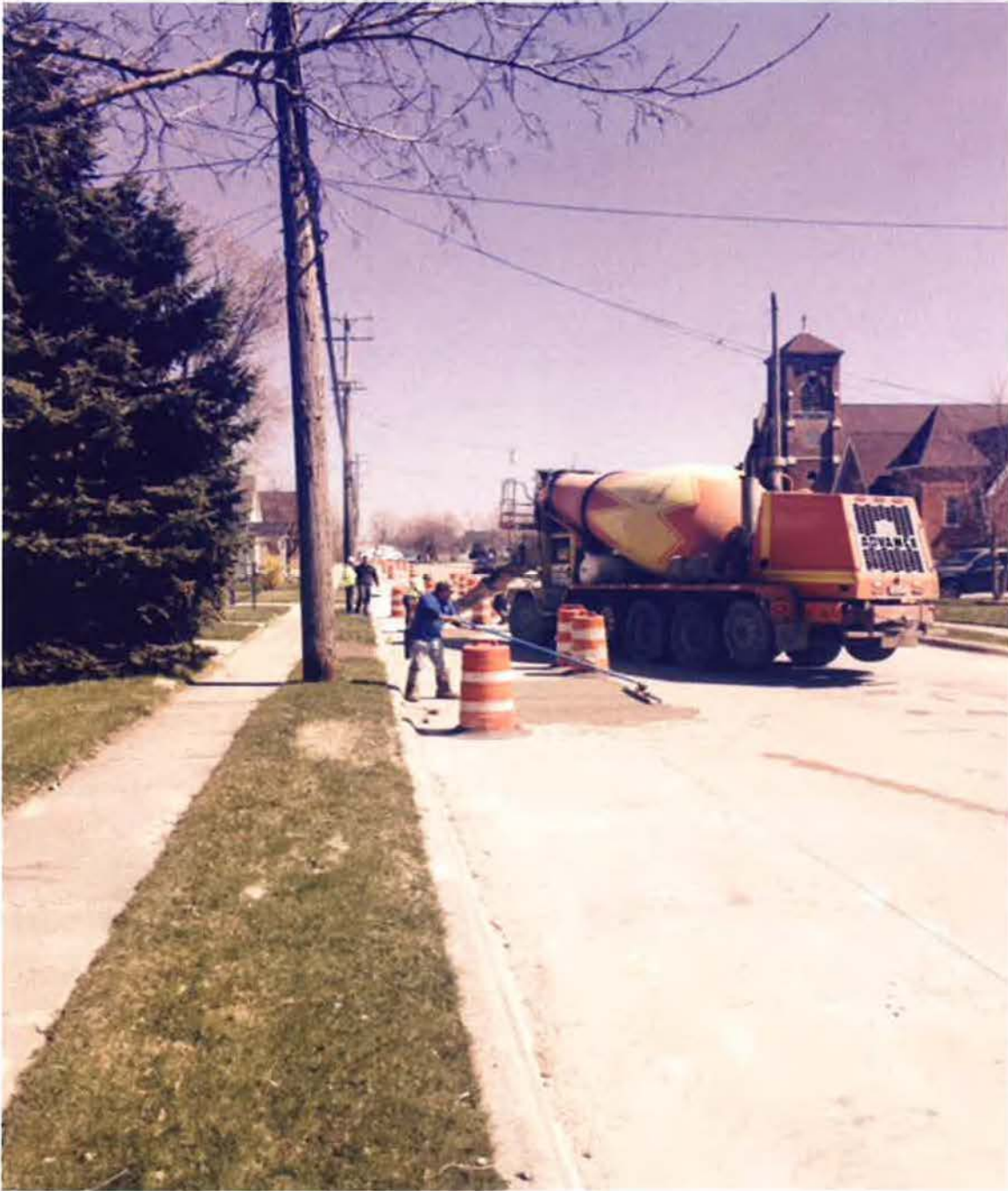
Concrete Road Repairs Rockwood
