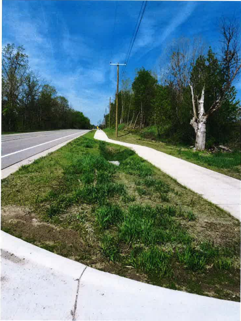
Half mile from Garfield Road – Looking west
