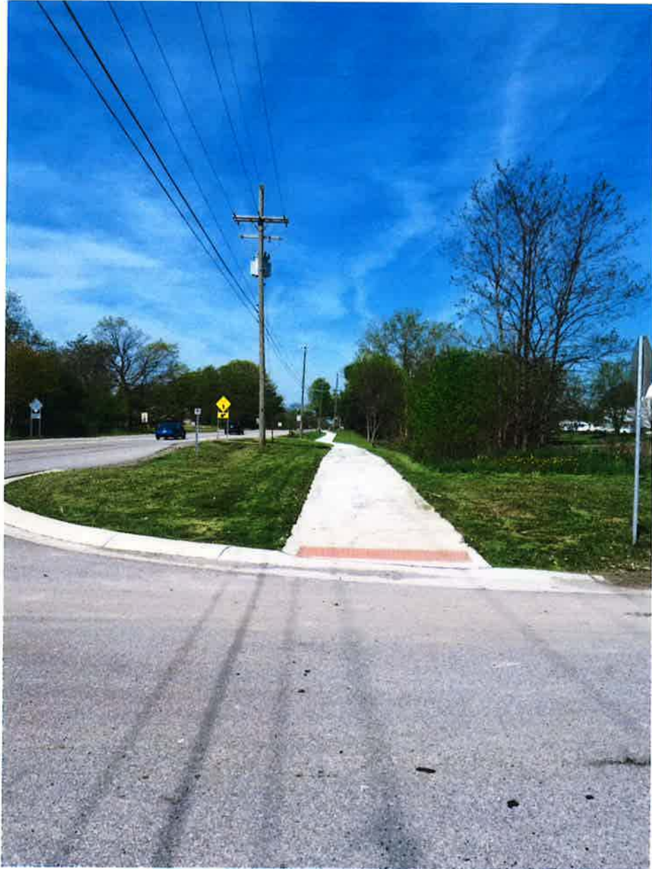
At Garfield Road – Looking west
