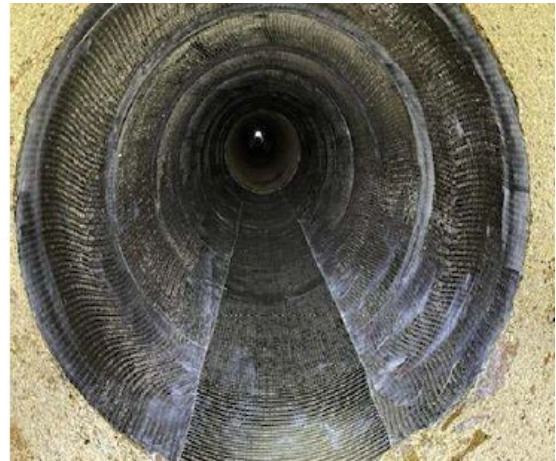
Figure 7: GFRP Install with cable for curing
