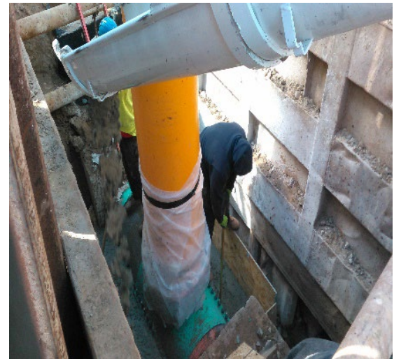
Figure 5: Line Stop Installation
