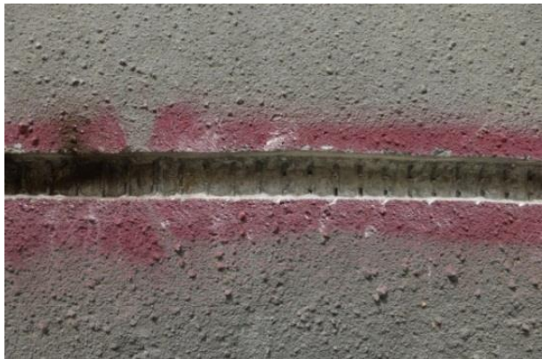
Figure 2: Cutting of Prestressing Wires
