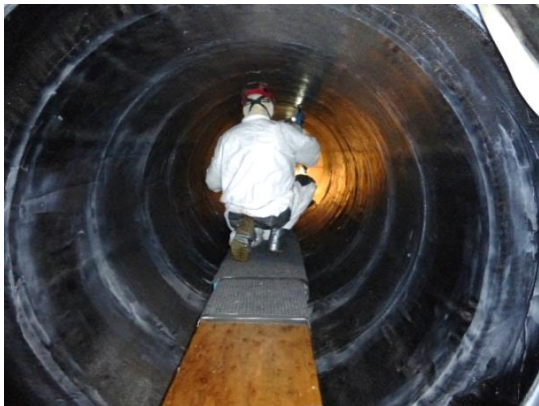
Figure 1: Installation of V-Wrap FRP Liner
