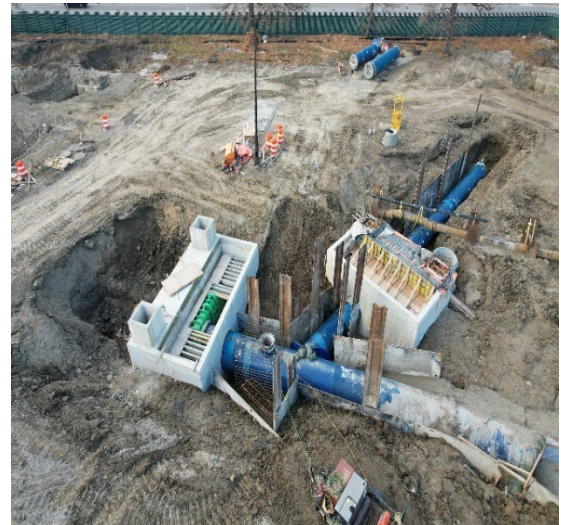
Figure 2: 48-inch WM and GV Installation
