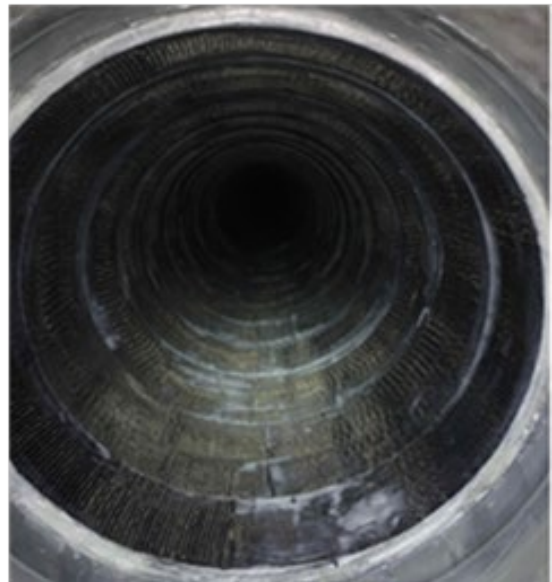
Figure 3: Initial Pipe Inspection
