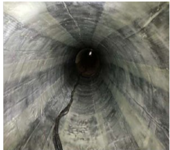
Figure 6: CFRP Partial Install
