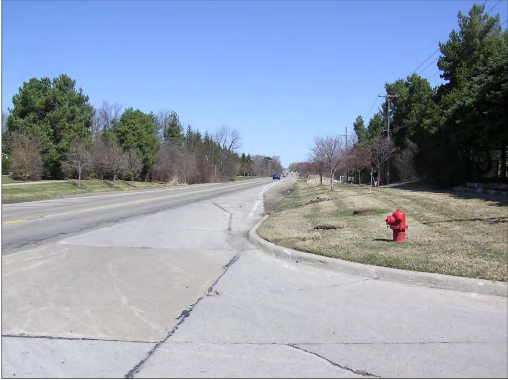
Figure 3. Looking North along East Side of Taft from White Pines
