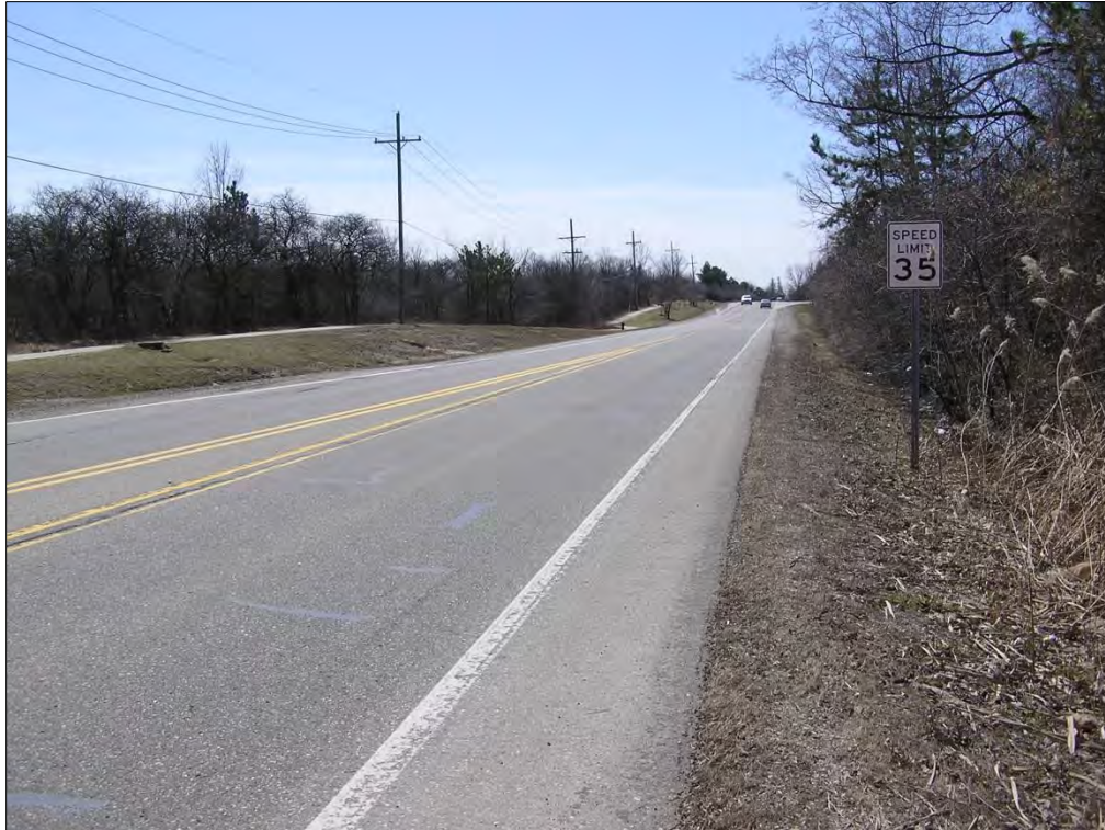
Figure 5. Looking South along West Side from Point Near Stadium Drive
