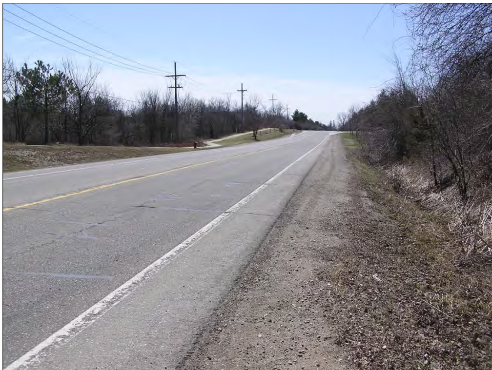
Figure 6. Looking South from Point where Shoulder Parking Becomes Possible
