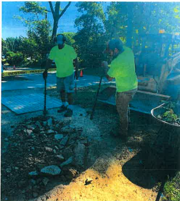
Path construction at Pondview Park
