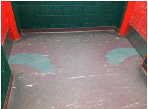
The existing lower level flooring is wearing away many spots and needs to be replaced. Flooring needs to cover completely or it can be a trip hazard and/or damage skate blades.
