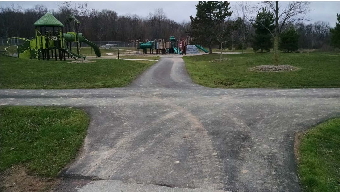
Rehabilitated Power Park Pathway intersection at north end of playground
