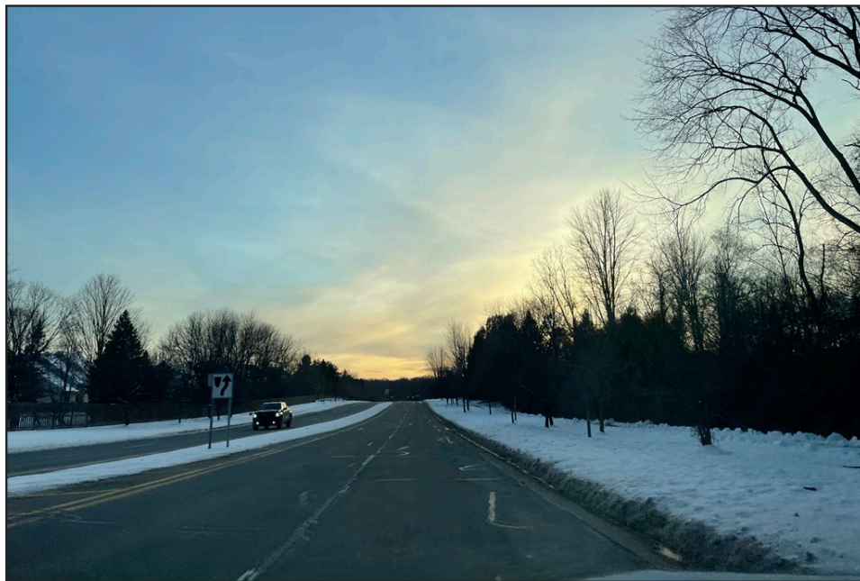
Novi Road Heading Southbound Near Old Novi Road. Source: OHM Advisors
