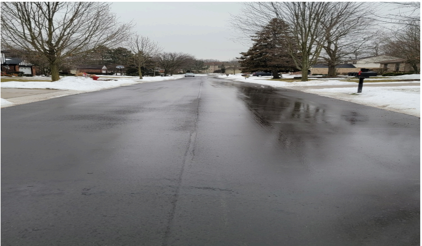
Orchard Ridge Subdivision – Harvest Drive – Completed
