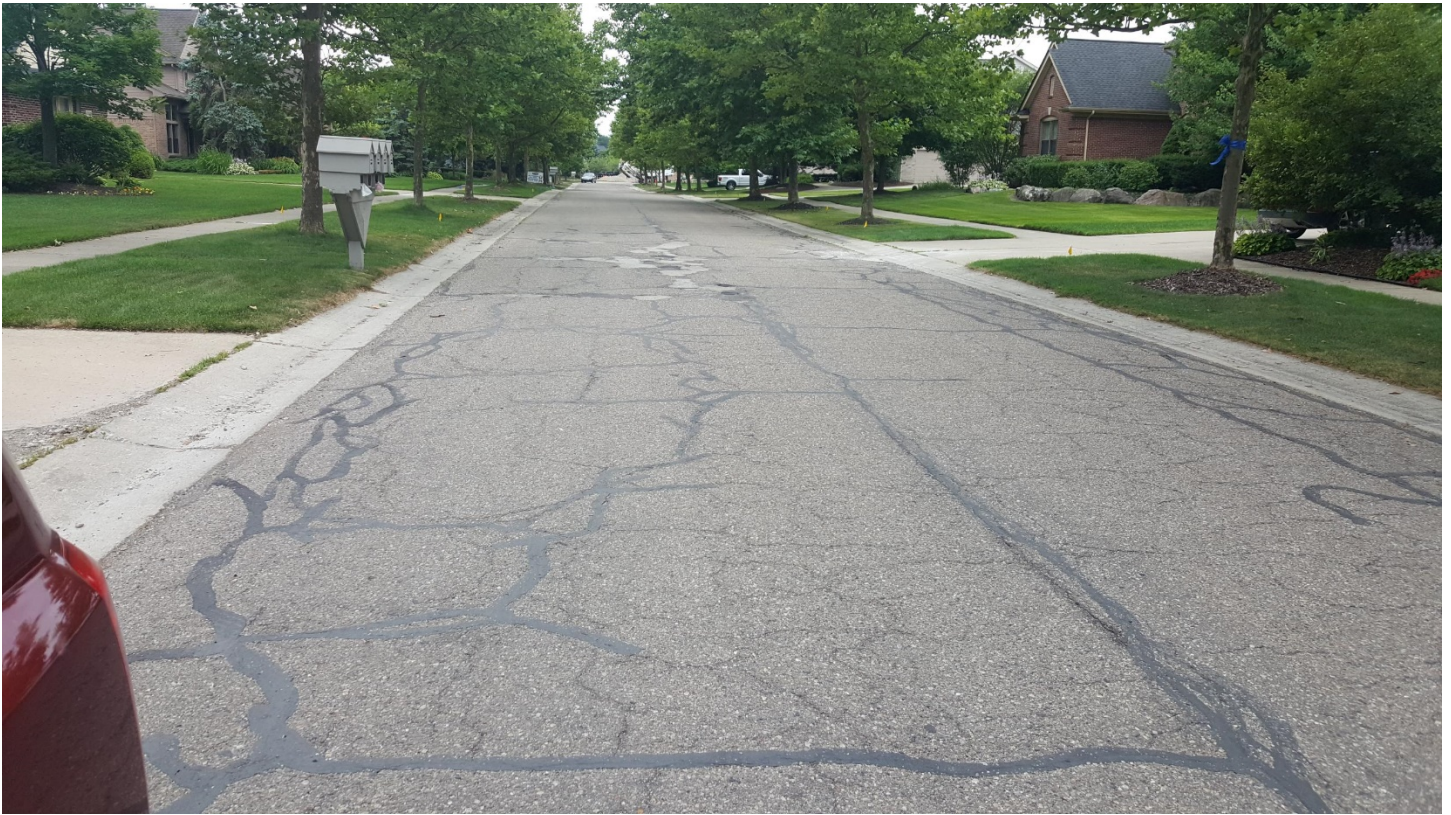
Greenwood Oaks Sub – Greenwich Drive – Pre-Construction
