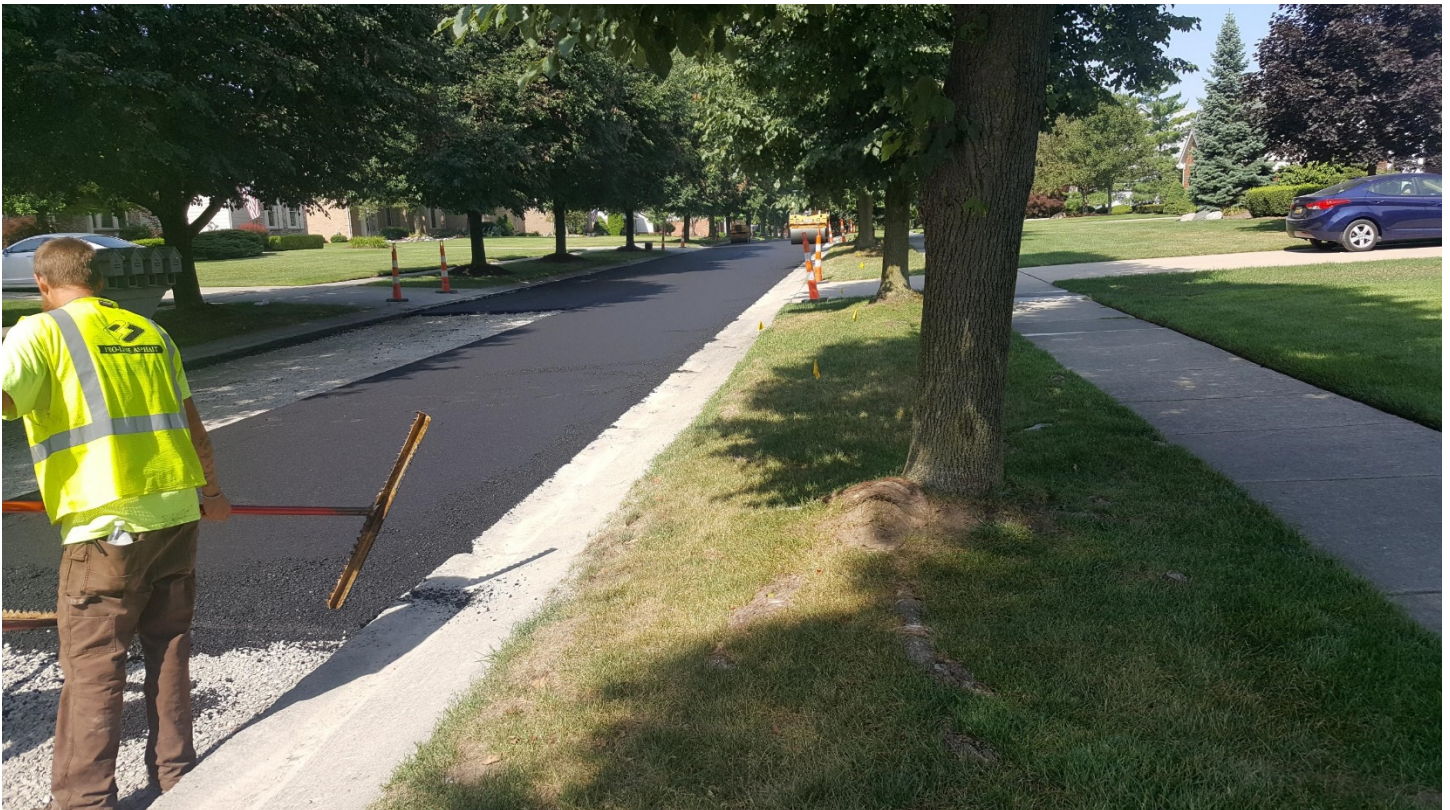
Greenwood Oaks Sub – Nantucket Drive – First Lift of Asphalt
