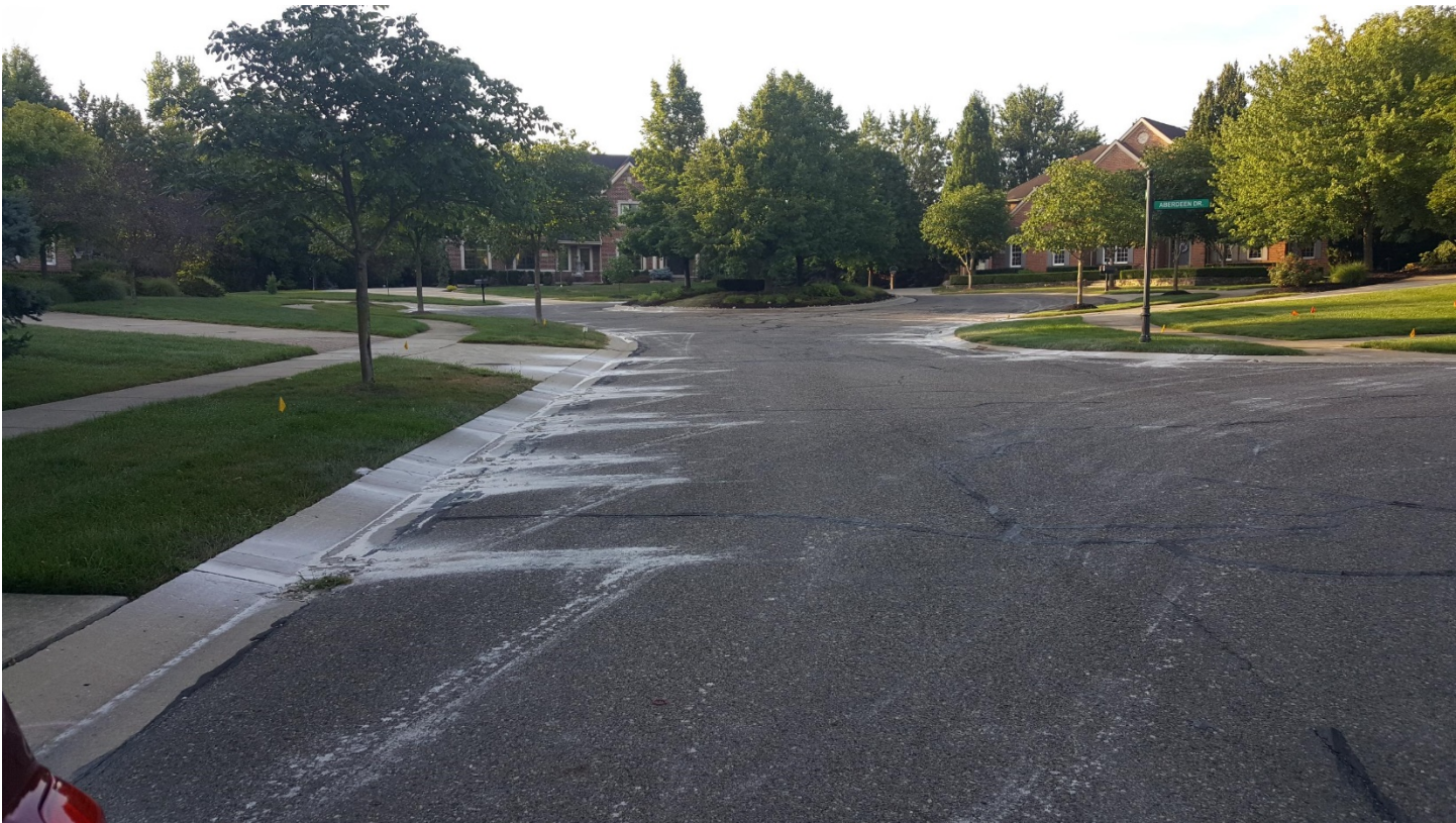
Greenwood Oaks Sub – Shilo Drive/Shilo Court – Pre-Construction
