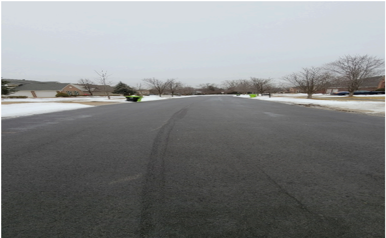
Brookhaven Subdivision – Myrtle Court off 10 Mile – Completed
