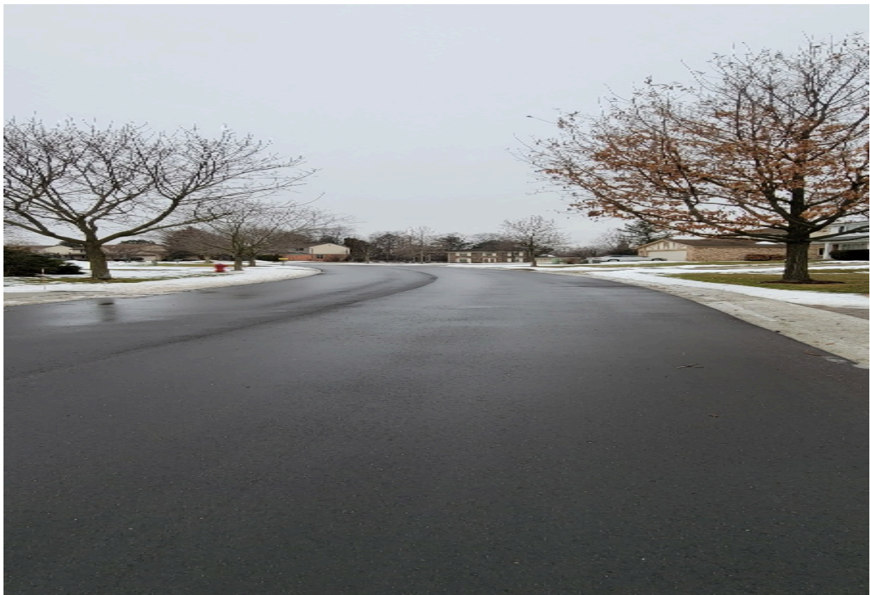
Orchard Ridge Subdivision – Hickory Grove - Completed
