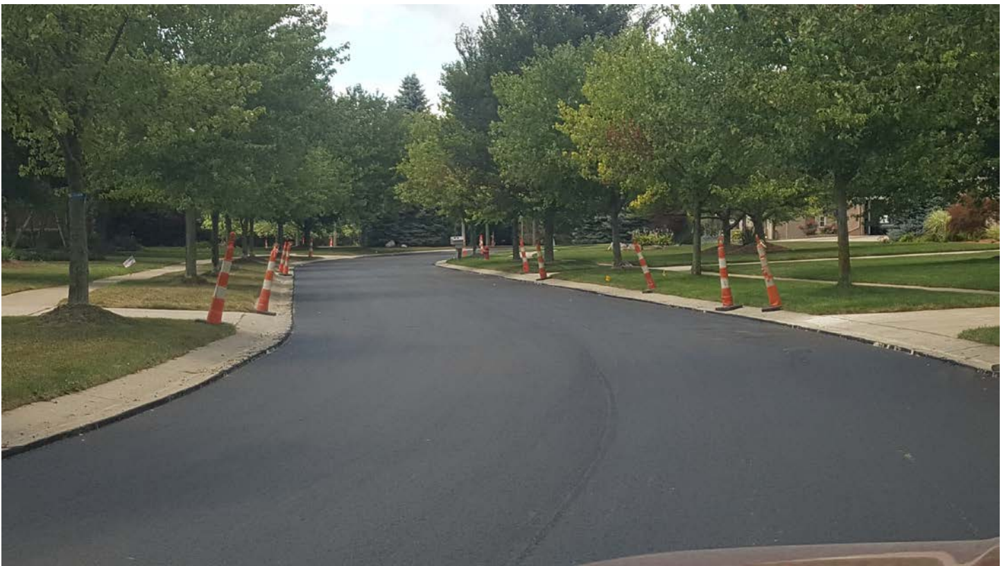
Greenwood Oaks Sub – Greenwich Drive – Completion of the first asphalt lift
