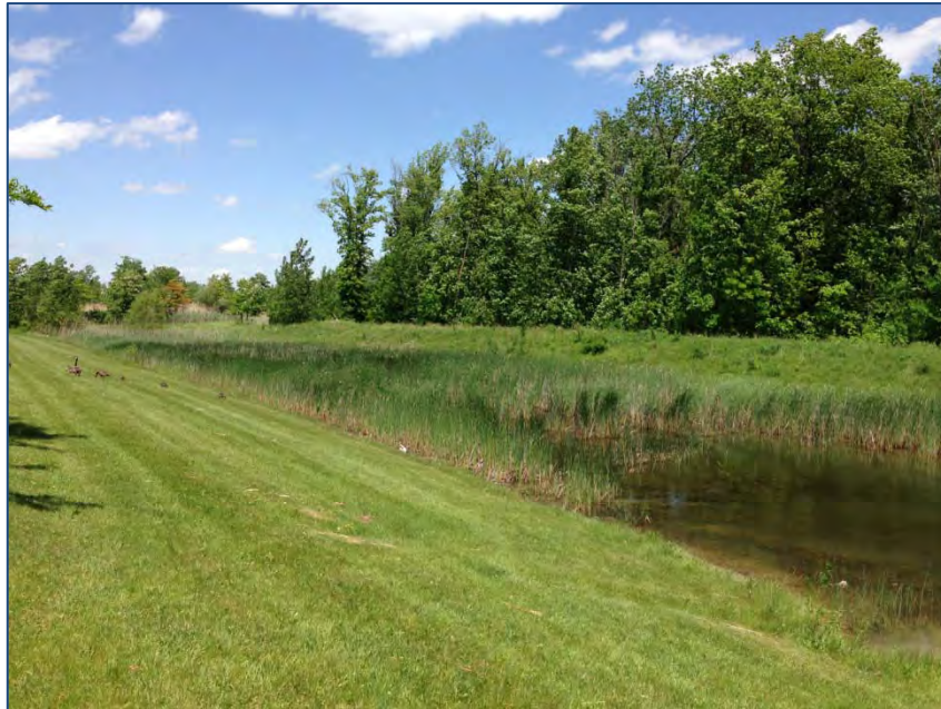
Photo 1. Looking north at west edge of existing detention basin. This basin to be replaced with proposed wetland mitigation area.
