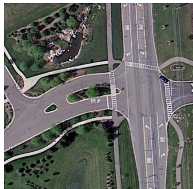
Raised Median at Glenwood Dr Entrance
