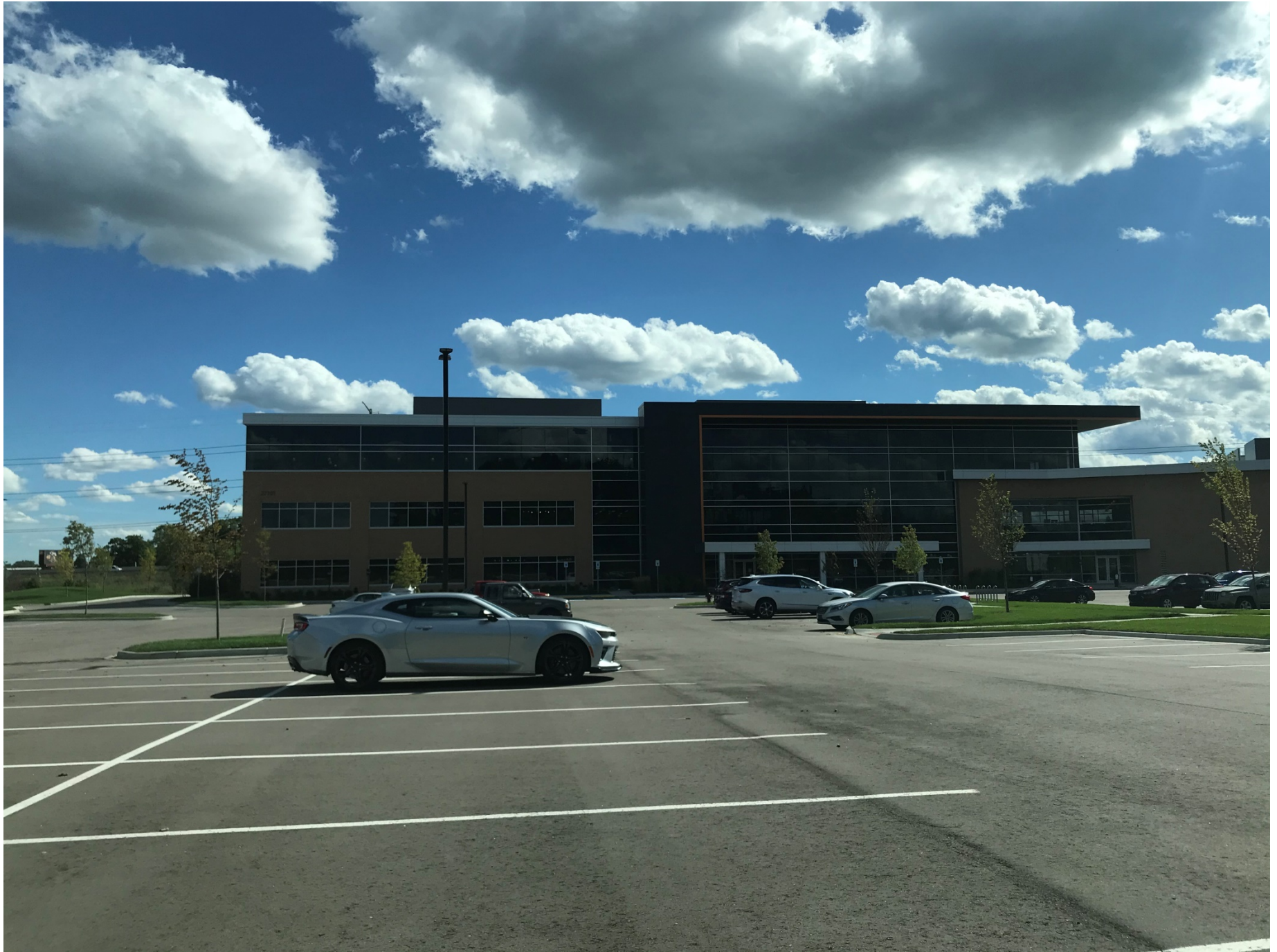
Figure 3: A123 Systems Headquarters
