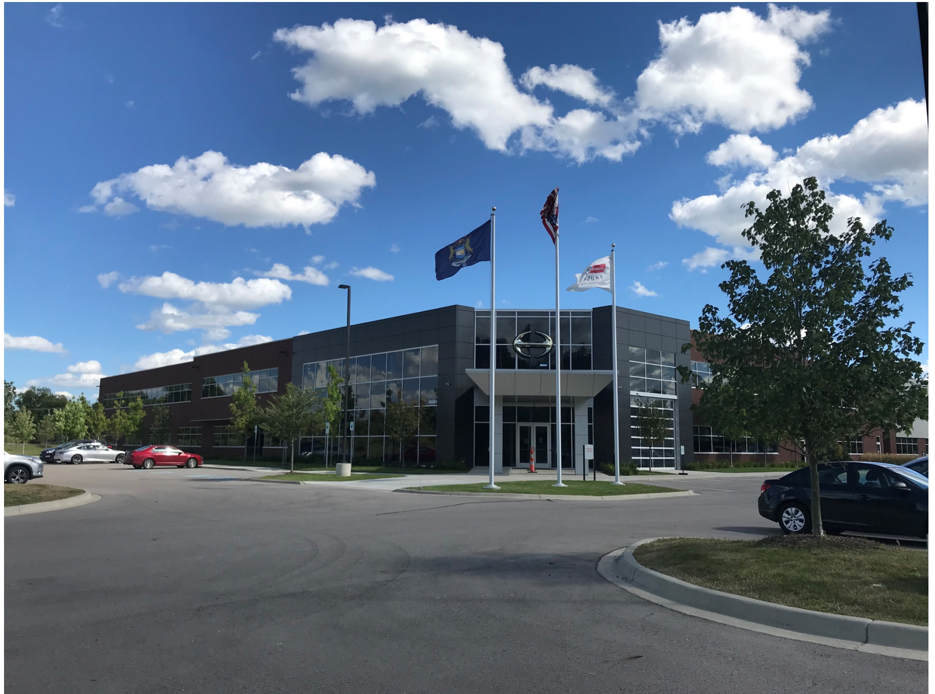
Figure 2: Hino Motors USA Headquarters
