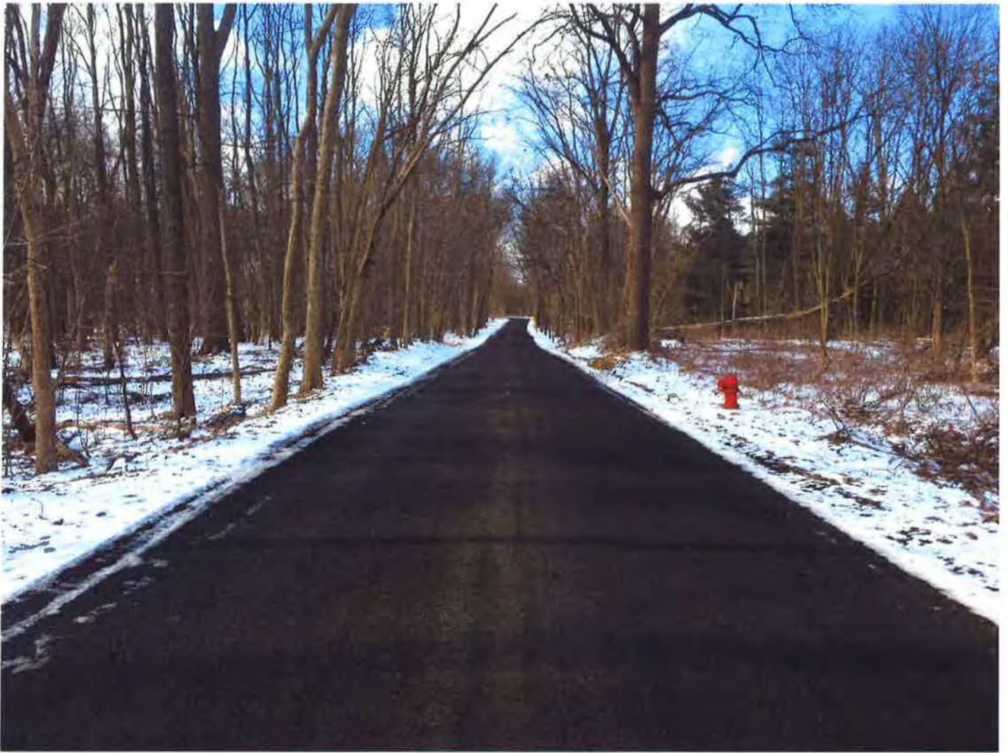
12 ½ Mile Road – Looking west towards Dixon Road
