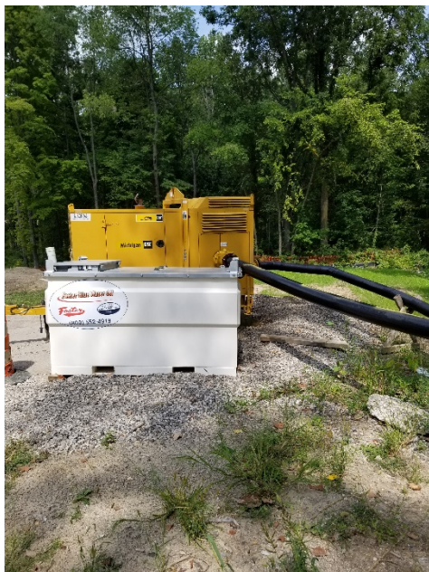
Pump used to direct water
