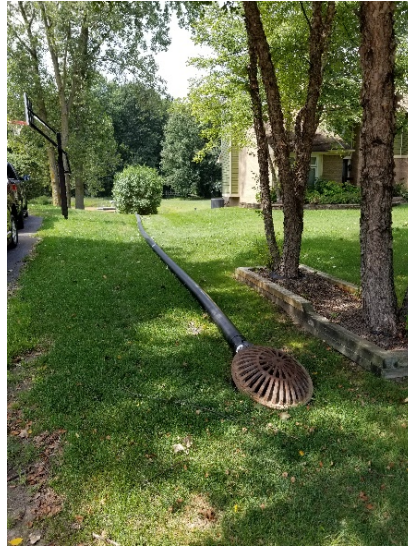
Piping along resident's yard
