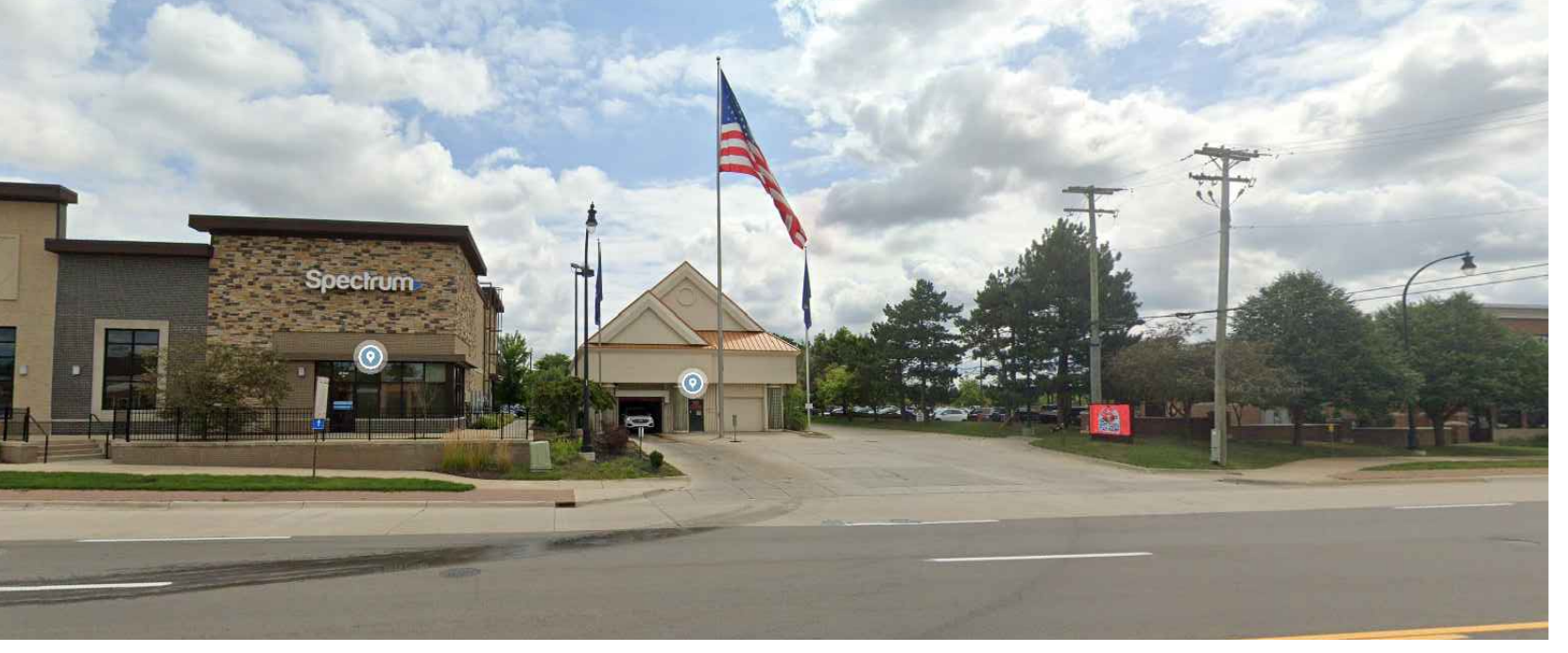
EXISTING CONDITION - SITE FRONTAGE NOT TO SCALE
