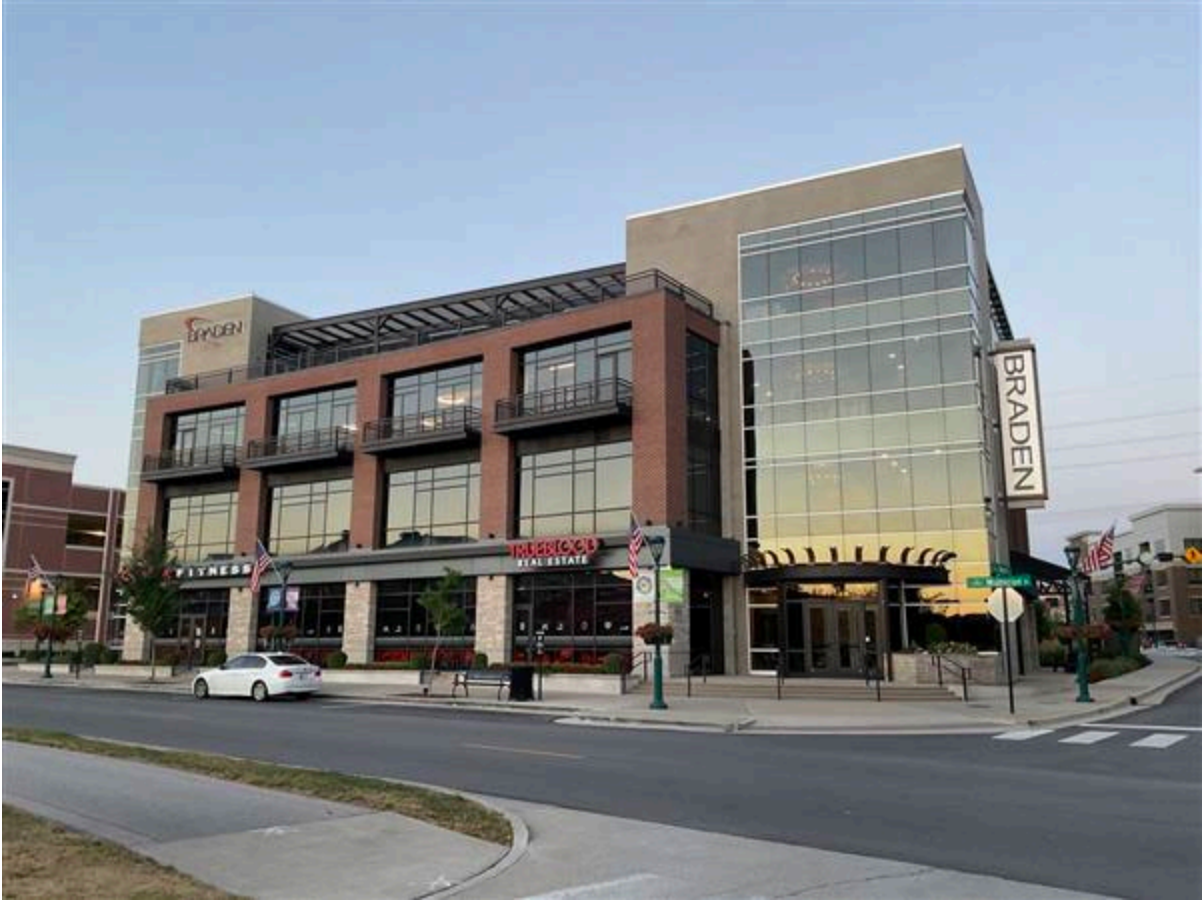
Commercial; occupants include business consulting, real estate, and fitness
