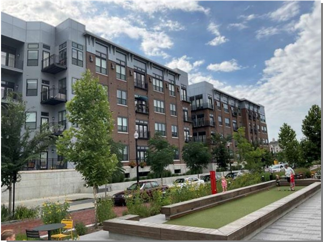
Left – mixed-use multi-family apartments
