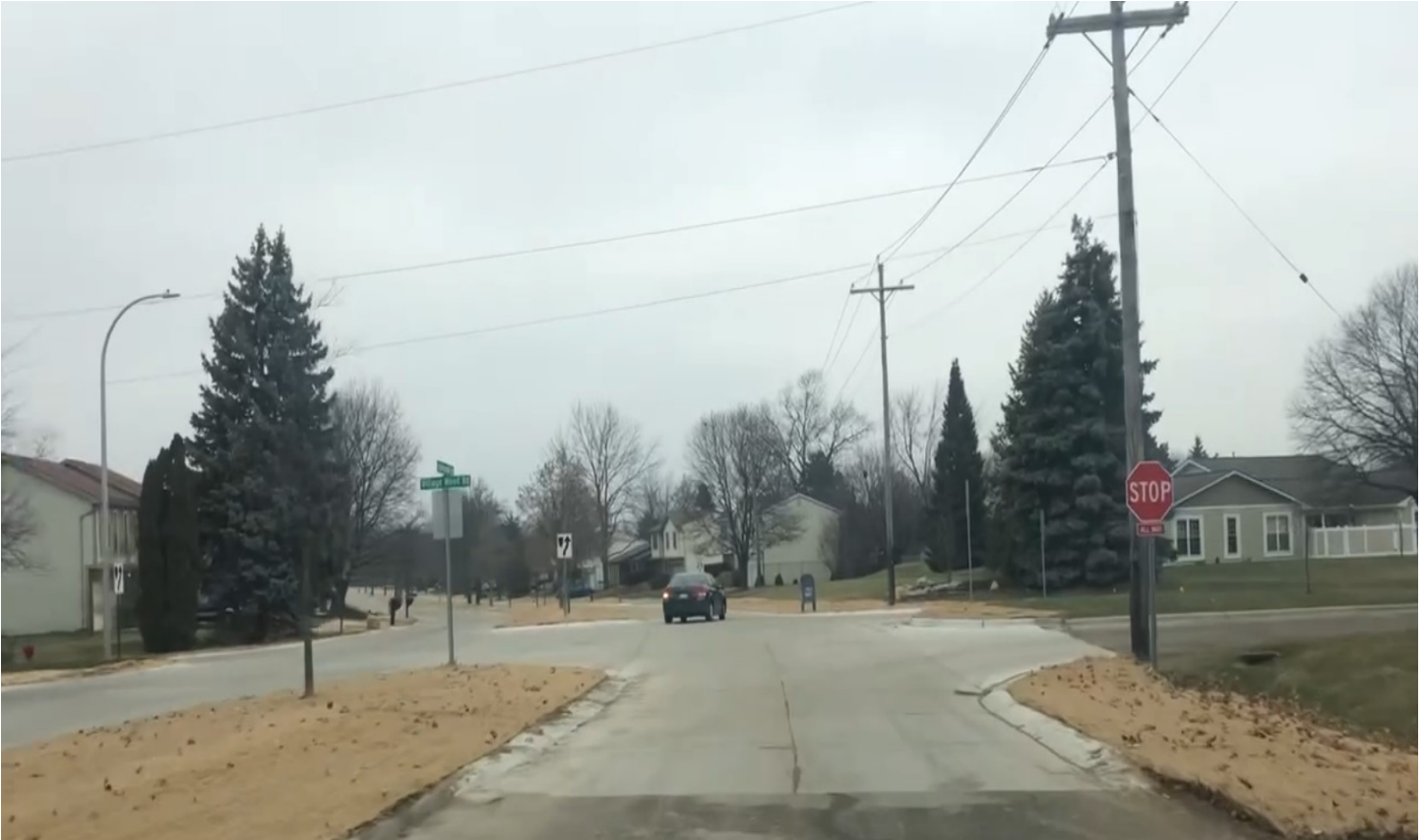
Cranbrooke Drive at Village Wood Road, looking north
