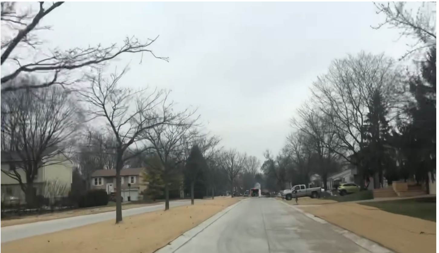
Cranbrooke Drive at Londonderry Drive, looking north on the northbound side
