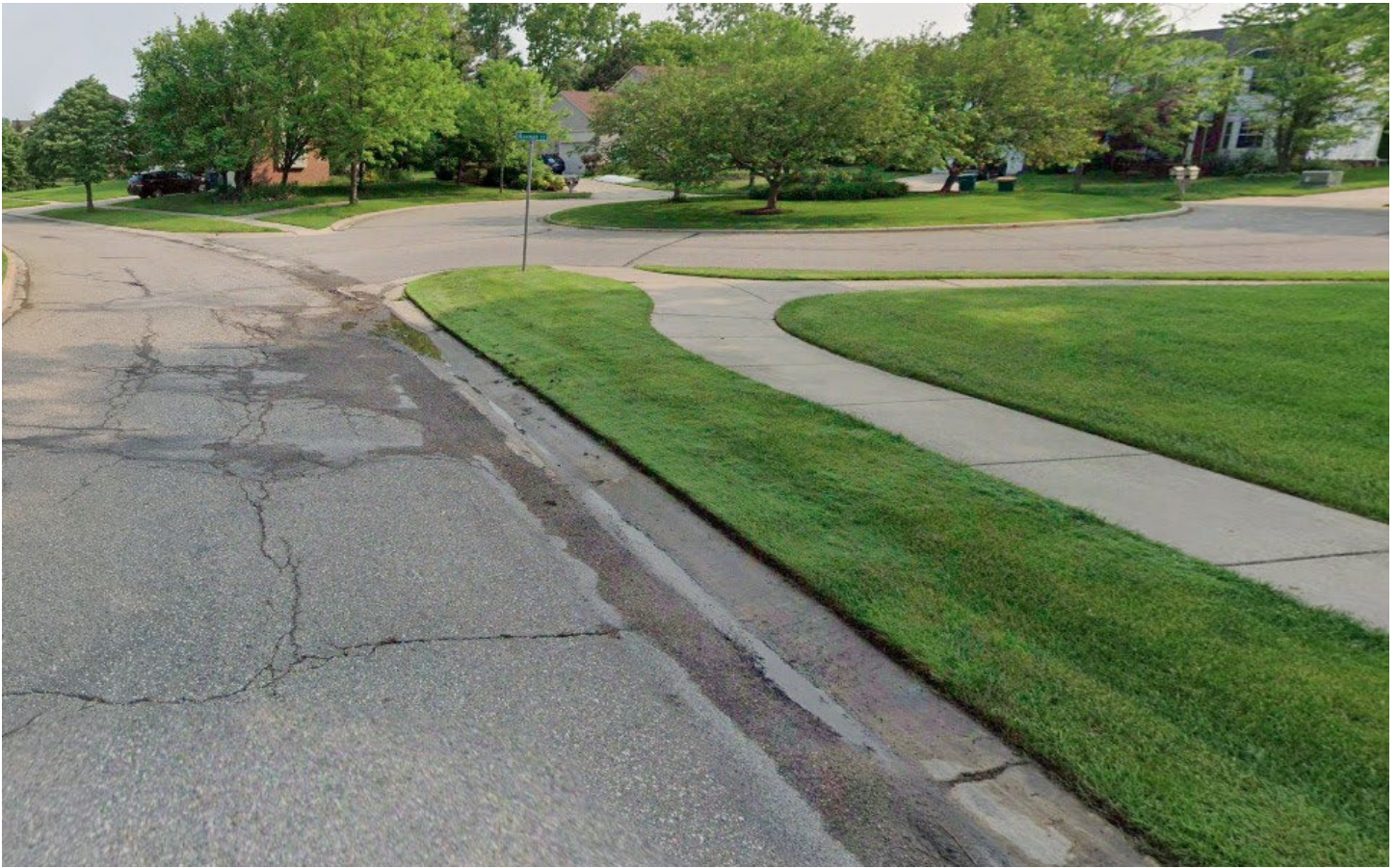
Before – Veranda Drive (Yerkes Manor), north of 8 Mile, looking north
