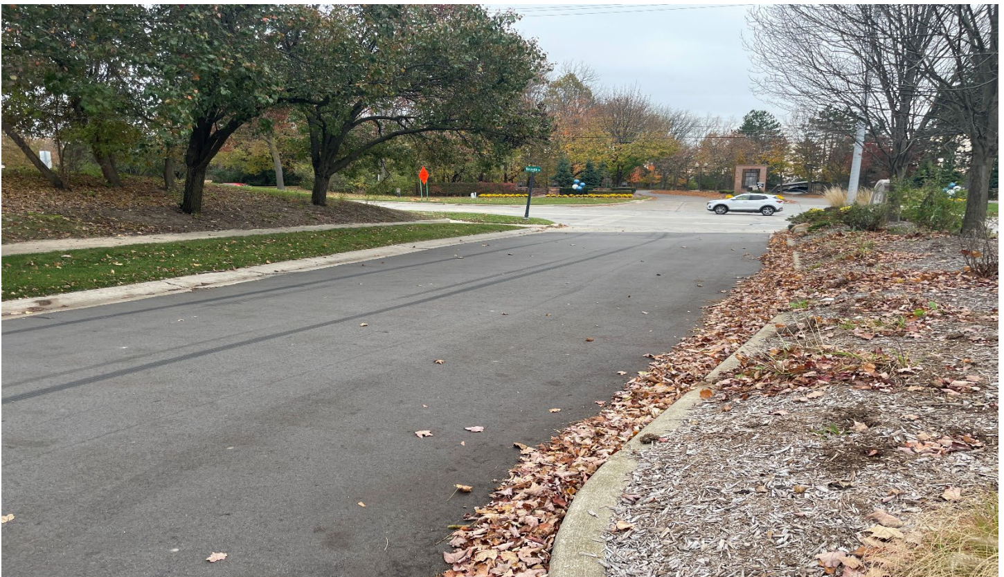
After – Veranda Drive (Yerkes Manor), north of 8 Mile Road, looking south
