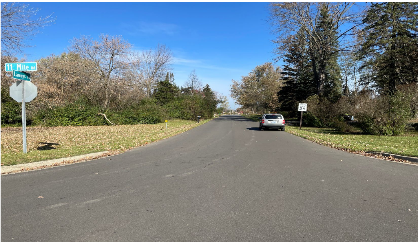
After – Lanny's Road, north of 11 Mile Road, looking north
