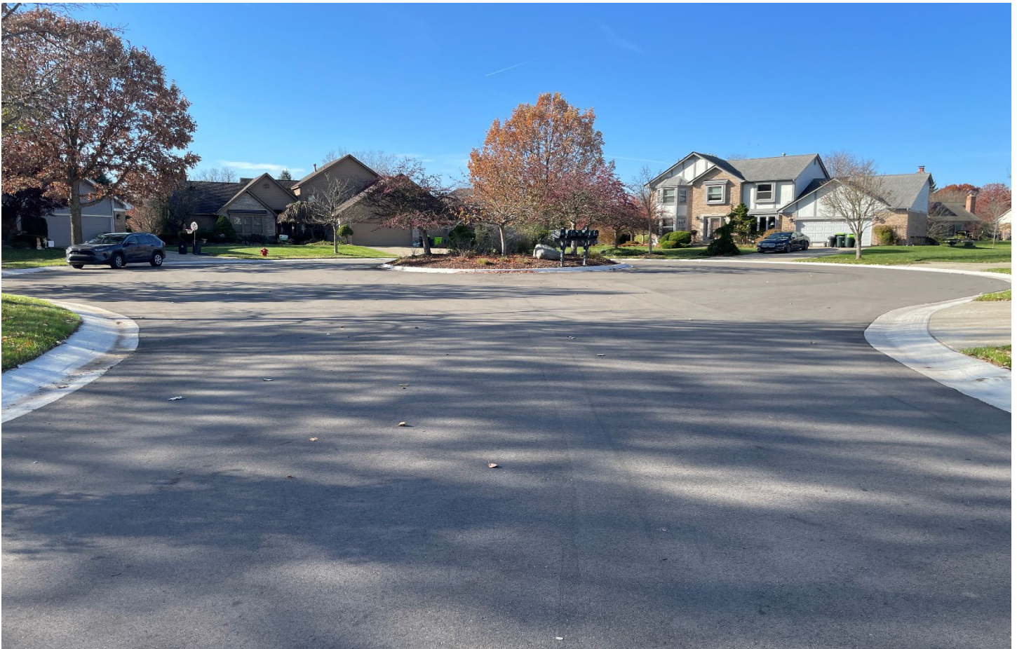
After – Stone Road, west of Buckminster Drive, looking west (Asphalt)
