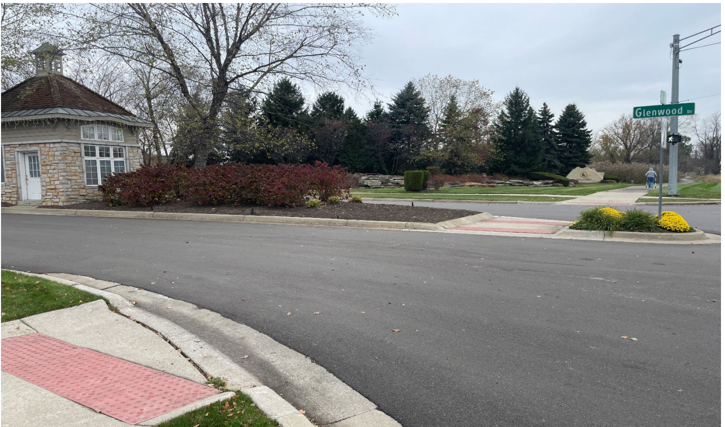
After – Glenwood Drive, west of Wixom Road, looking north
