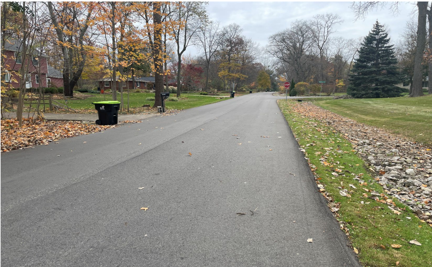
After – Galway Drive, east of Connemara Drive, looking west
