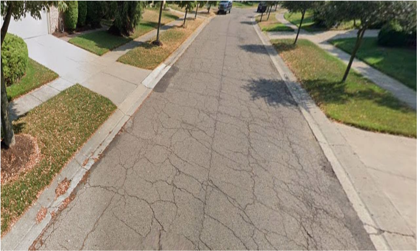
Before – Groveland Road (Lochmoor Village) looking north
