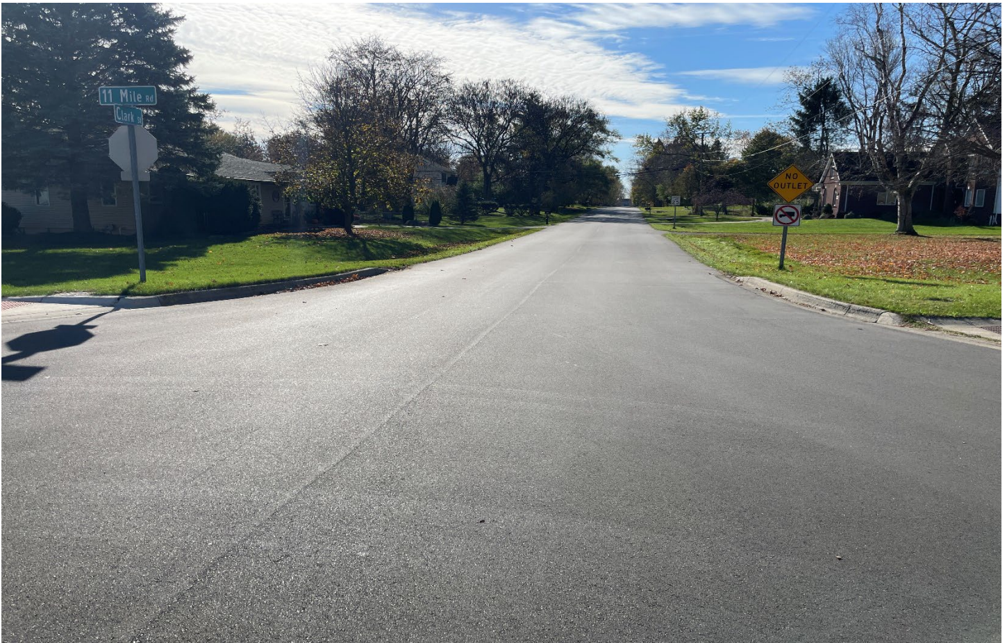
After – Clark Street, north of 11 Mile Road, looking south
