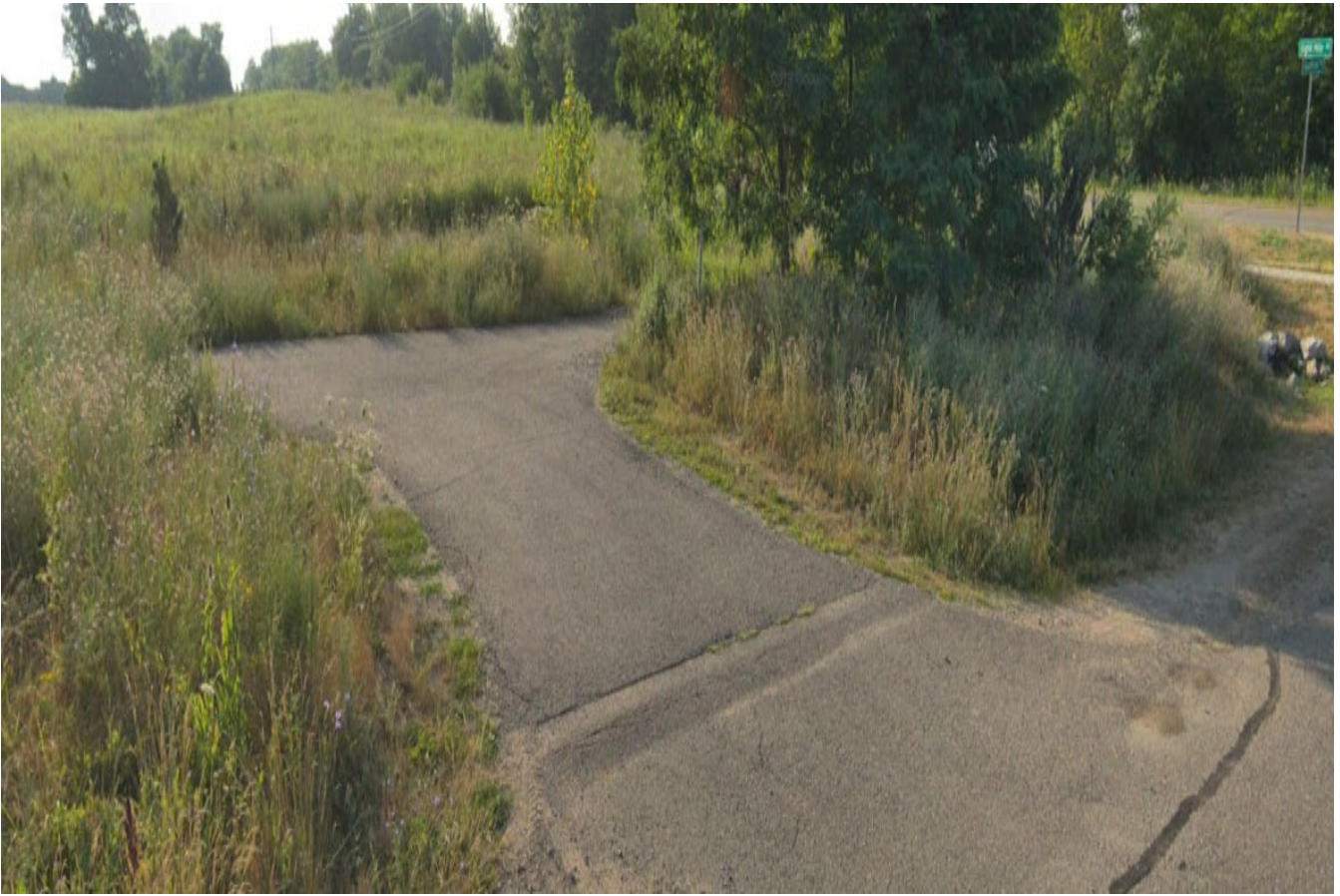
Before – S.A.D. 170A Pump Station prior to construction
