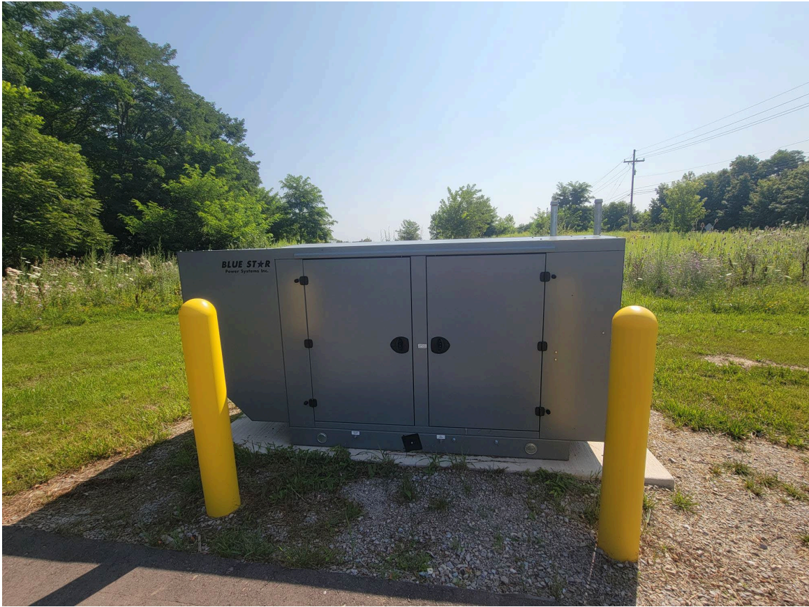
After – Placement of generator pad and natural gas generator
