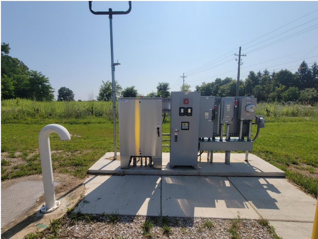
After – Placement of Pump Station equipment
