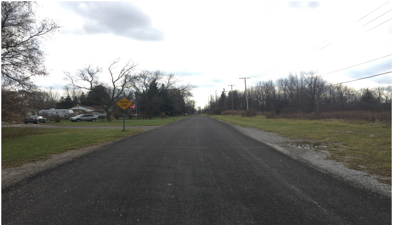
Taft Road – Looking south from 12 Mile Road
