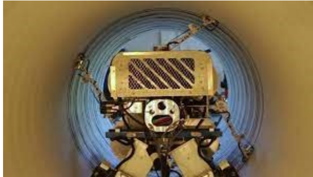
Figure 20: SippTech MICP Liner Installation (Photo Courtesy of SippTech Website)
