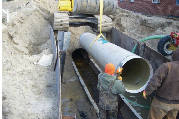
Figure 4: Hobas Pipe Installation (Photo Courtesy of Hobas Pipe USA Website)
