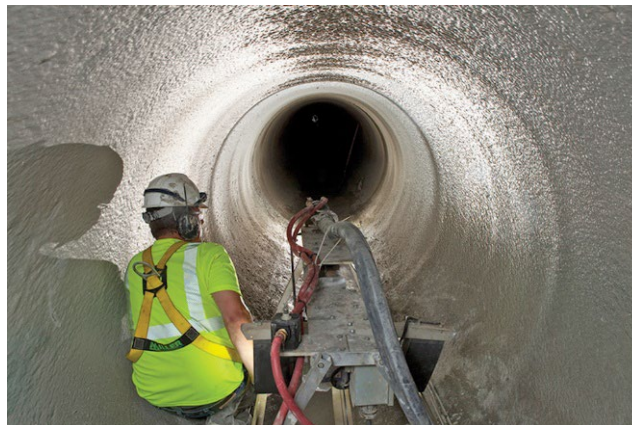
Figure 21: Spray-On Liner/Coating Installation (Photo Courtesy of Municipal Sewer & Water Magazine Website)
