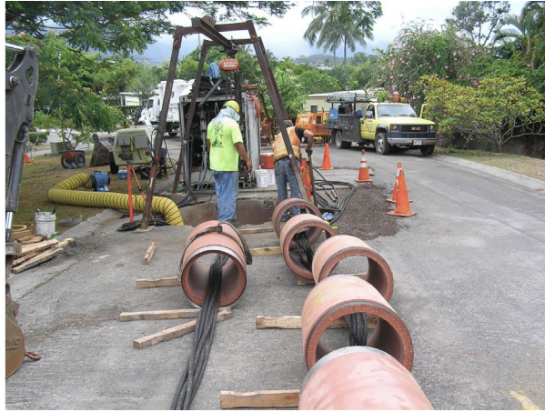
Figure 11: Logan Clay Pipe Installation (Photo Courtesy of Logan Clay Pipe Presentation)
