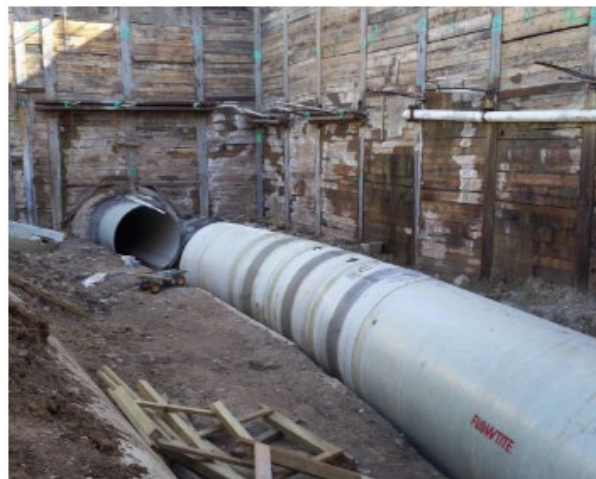
Figure 3: Thompson Flowtite Pipe Installation (Photo Courtesy of Thompson Pipe Group Presentation)
