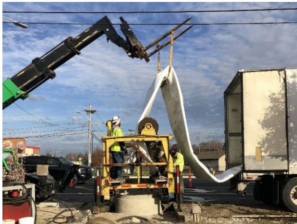
Figure 17: CIPP Felt Liner Inversion during Elizabeth Lake Road Sinkhole Sewer Rehabilitation
