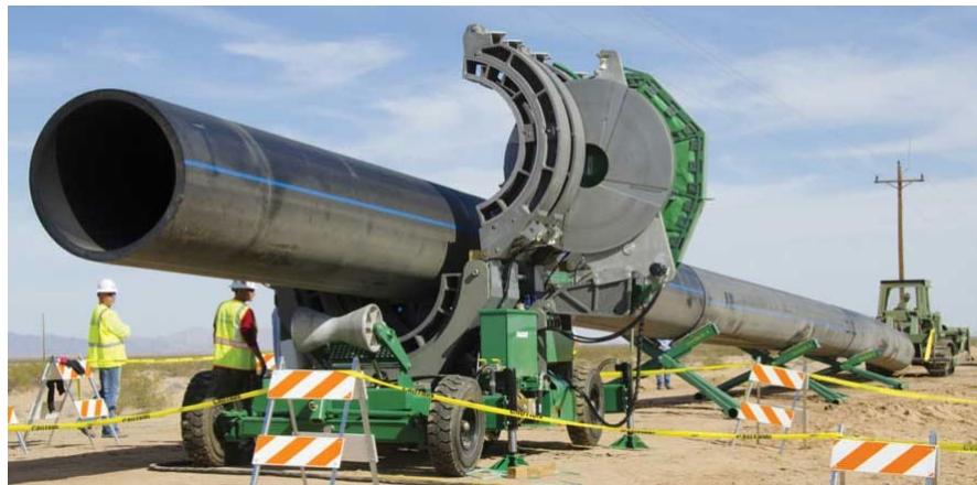
Figure 8: Fusion-Welded HDPE Pipe (Photo Courtesy of Trenchless Technology Magazine Website)
