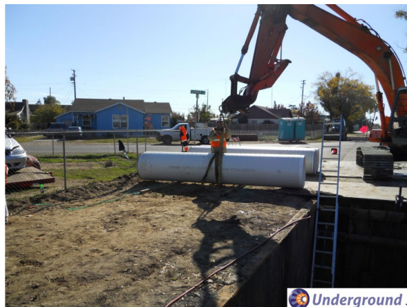
Figure 13: Vylon PVC Slip-Liner Installation (Photo Courtesy of Underground Solutions Presentation)
