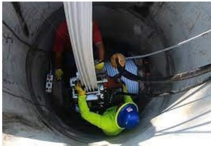
Figure 14: Sekisui SPR-EX Liner Installation (Photo Courtesy of Sekisui Website)
