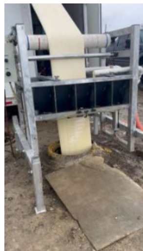
Figure 19: RigidSeal Pipeline Installation (Photo Courtesy of RigidSeal Presentation)
