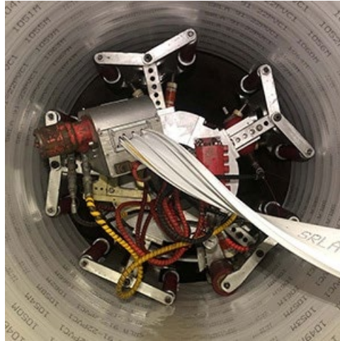
Figure 15: Sekisui SPR-TF/RO Liner Installation (Photo Courtesy of Sekisui Presentation)
