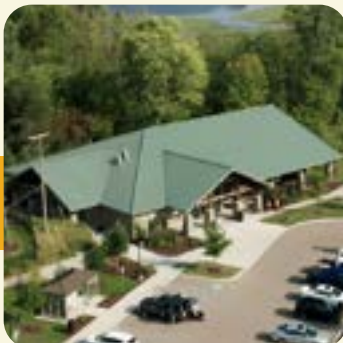
Lakeshore Park Building & Renovations
