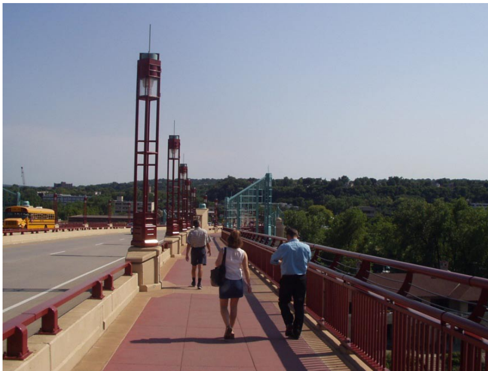
Wabasha Street Bridge in St. Paul Minneapolis
