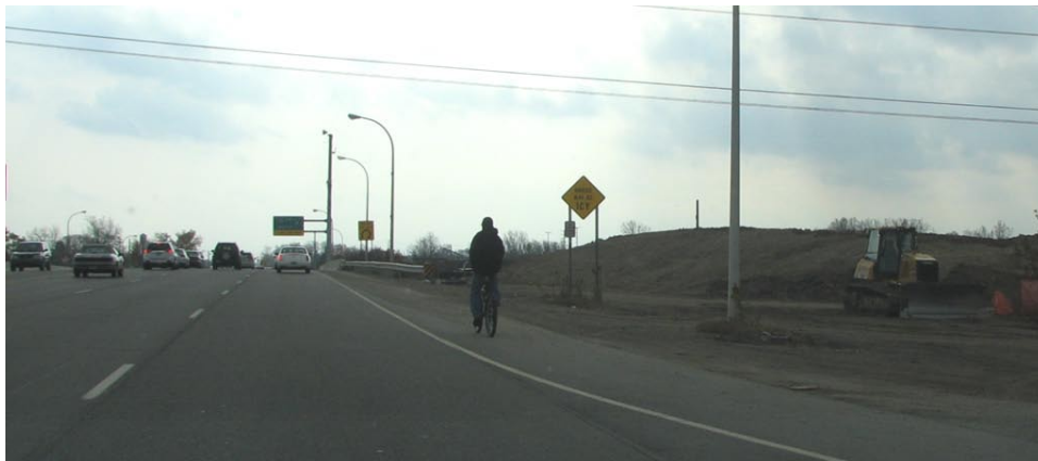
Existing conditions for the Novi Street overpass
