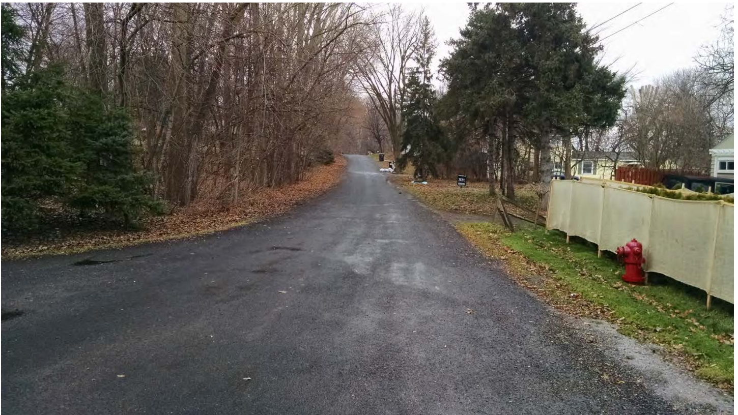
2014 Chip Seal Program – Looking South Along Shawood Drive at Crown Drive.
