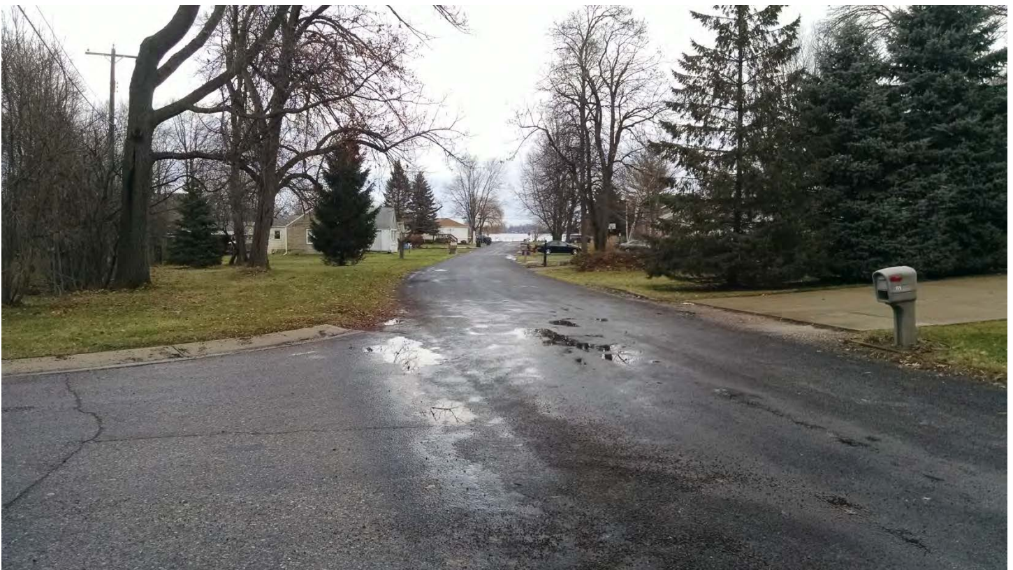
2014 Chip Seal Program – Looking North Along Buffington Drive at Lilley Trail.
