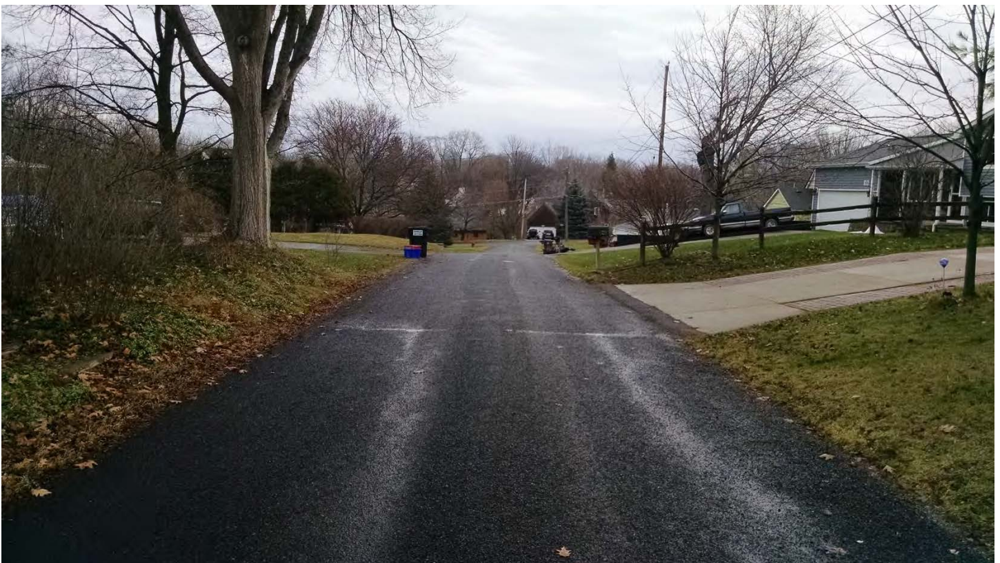
2014 Chip Seal Program – Looking Northeast Along Shamrock Hill towards Crown Drive.
