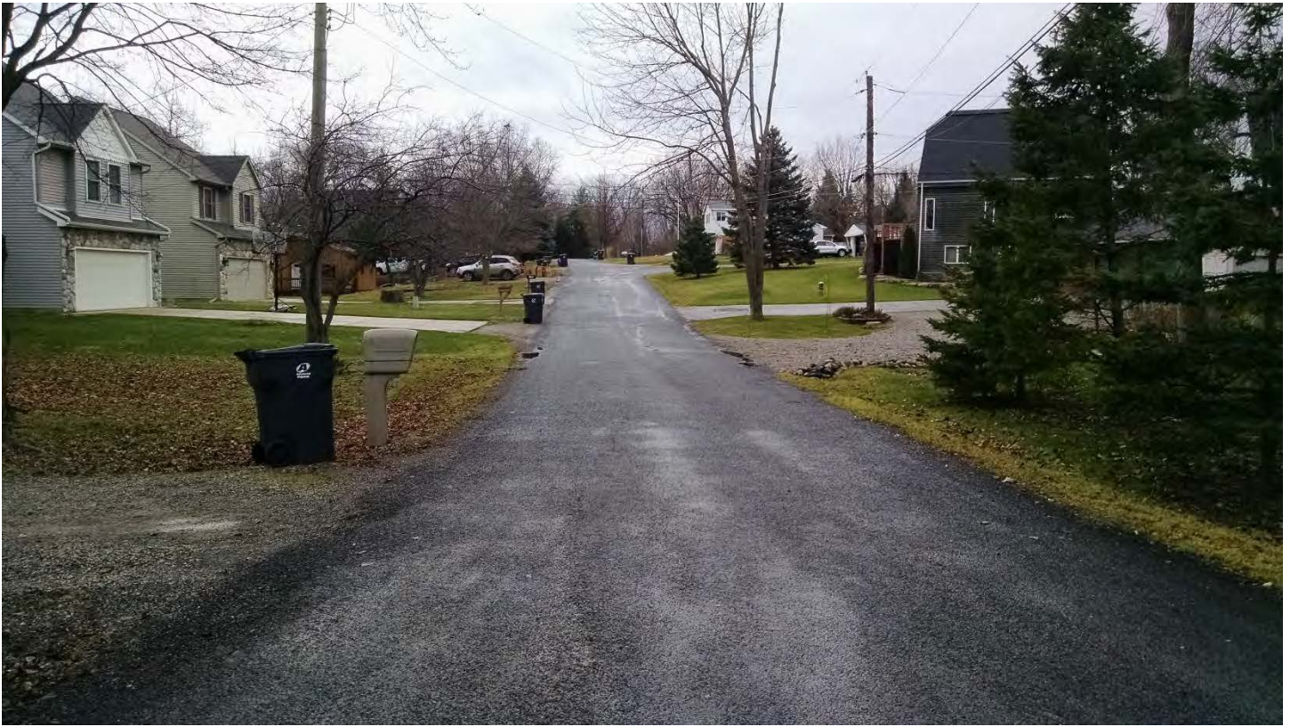
2014 Chip Seal Program – Looking South Along Crown Drive from Shawood Drive.
