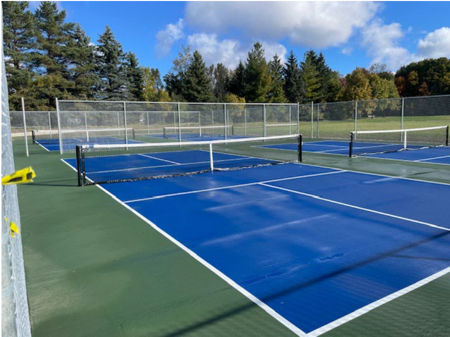
After – New courts complete
