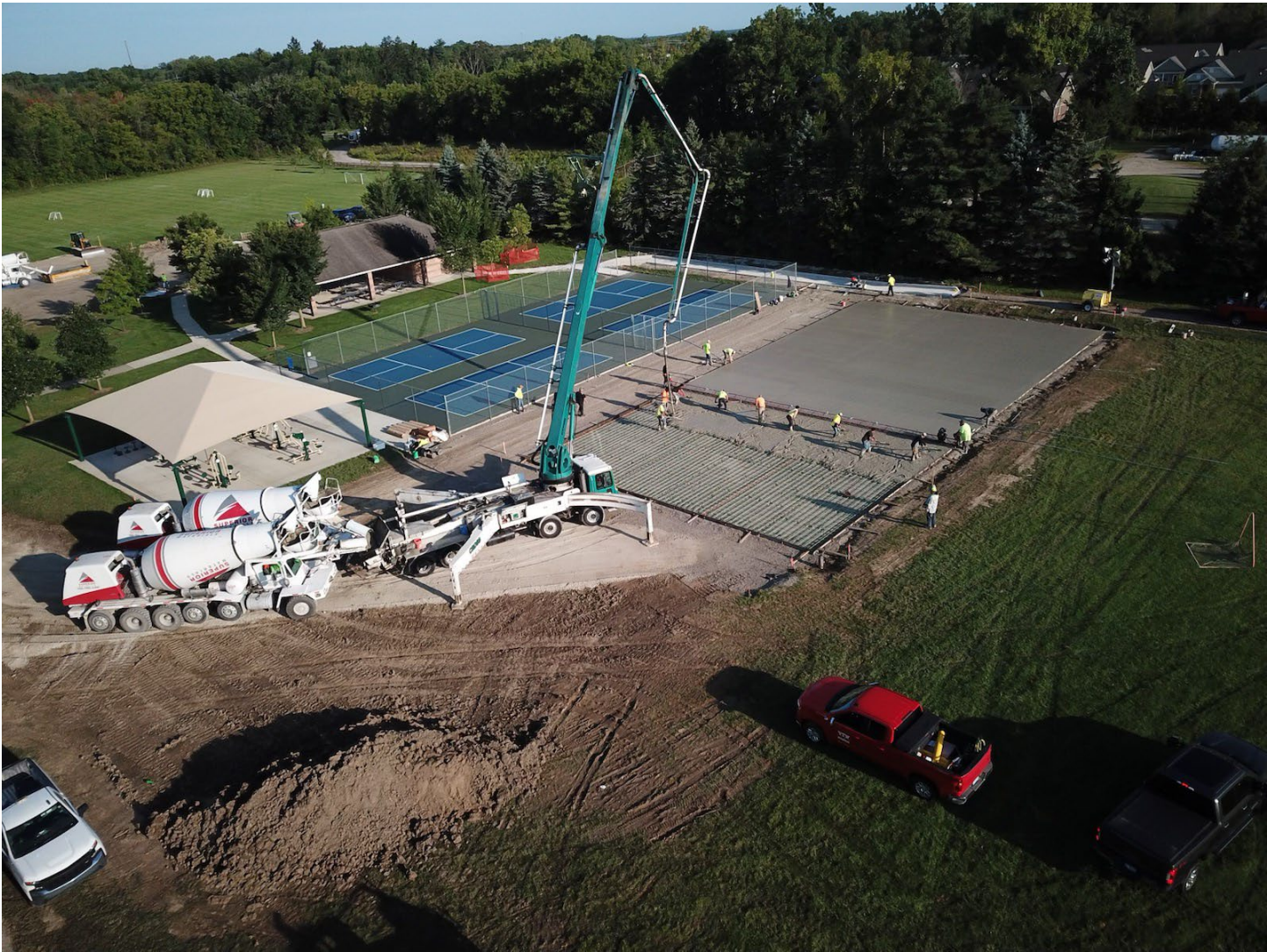
During – Pumping concrete for new courts
