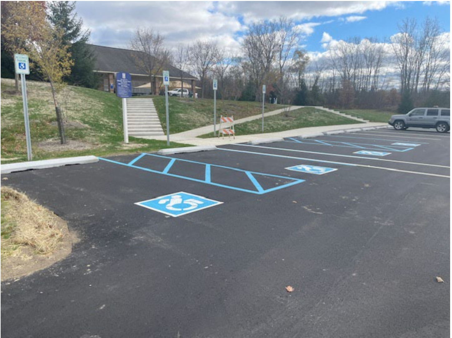
After – Looking east at new parking lot expansion and concrete stairs
