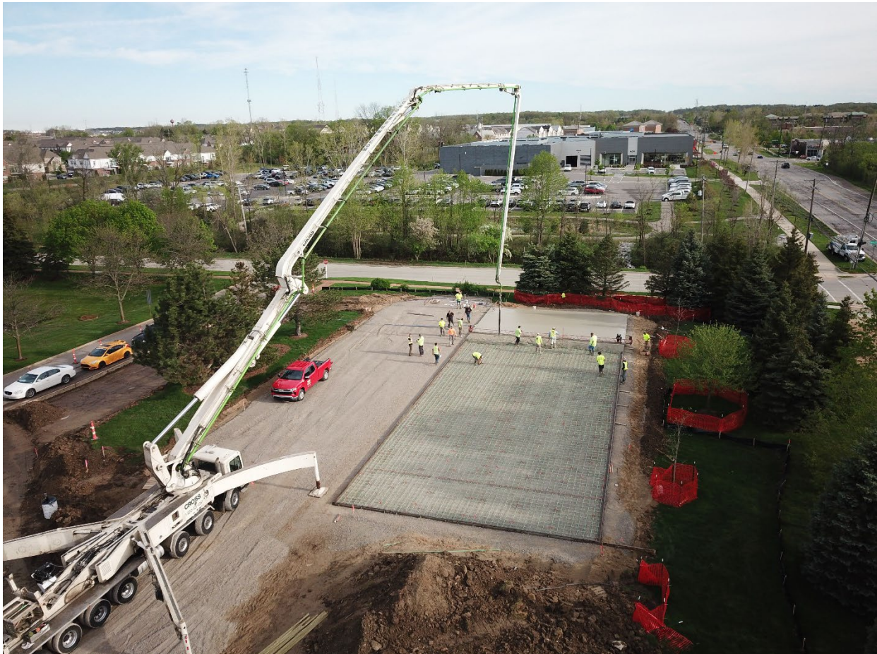
During – Pumping concrete for new courts
