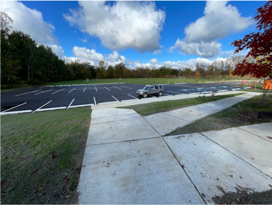
After – Looking west at new parking lot expansion and concrete stairs
