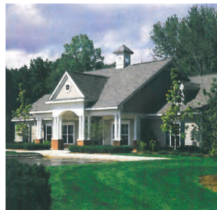
HARRISON COVE / Harrison Twp. / Michigan / Harrison Cove with it's state-of-the-art clubhouse provide It's residents with olympic sized pool work-out center and business center. Starter home condominiums with one-car attached garages.
