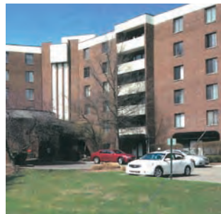
CLAYMOOR / Southfield / Michigan / Midrise apartments with convenient commercial amenities on the main floor: Clubhouse, pool and covered garage. Southfield's soundproof premier apartment community.
