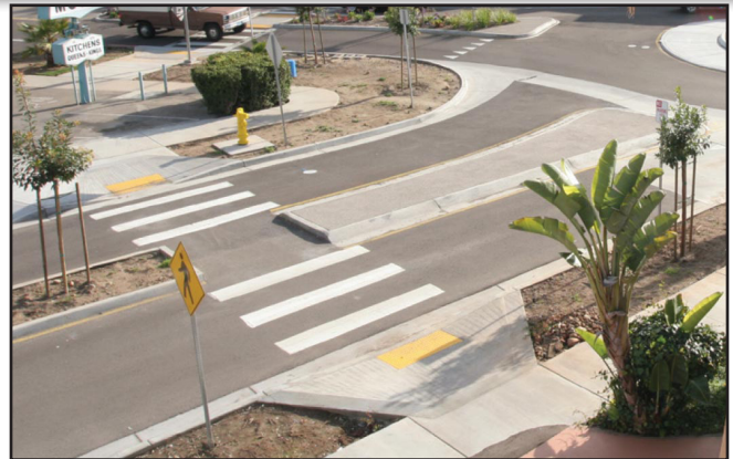
Improving the visibility of crosswalks alerts drivers to the potential for pedestrians. Source: FHWA
