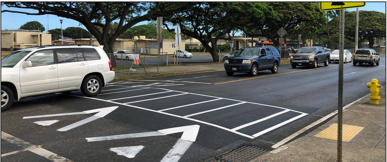
Raised crosswalk sat intersection force vehicles to slow down and make pedestrians more visible. Source: FHWA
