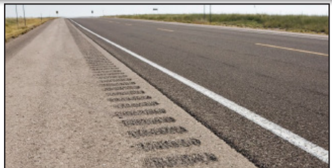
Rumble strips alert drivers to lane changes. Source: FHWA
