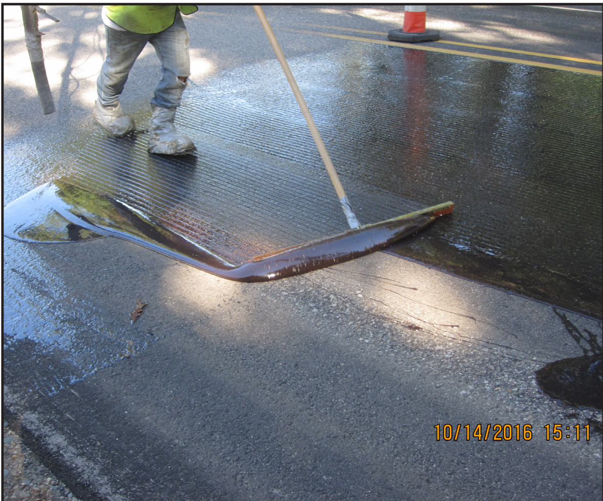
High friction surface treatment on Clarkston Road. Source: RCOC
