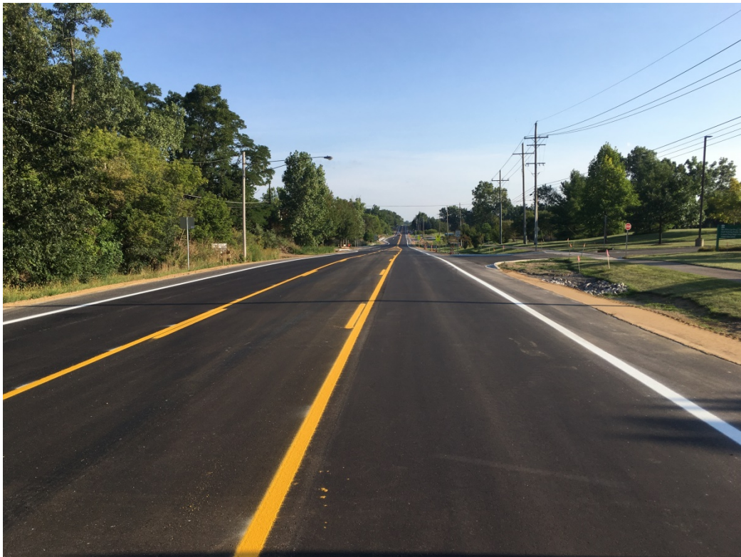
Southbound lane of Taft Road looking south from Novi Meadows Elementary
