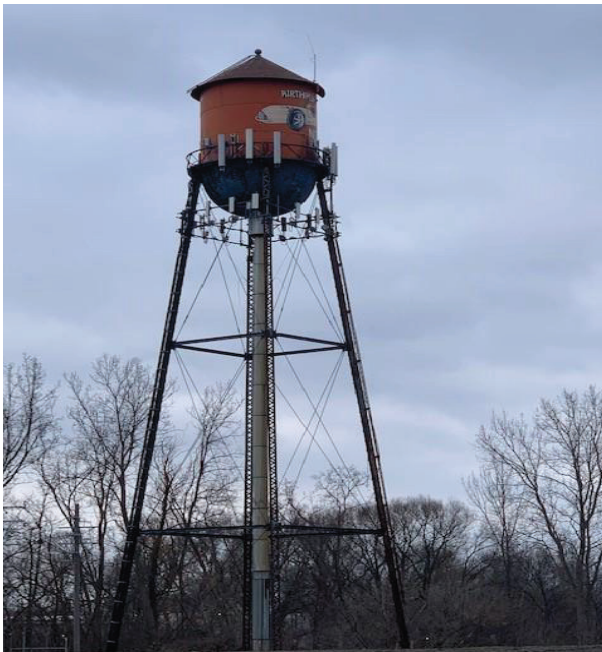
Total Steel Structure
