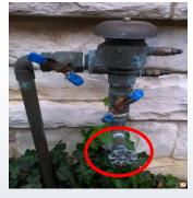
Testable Pressure Vacuum Breakers (PVB) for use on typical lawn sprinkler systems under continuous pressure (note unprotected hose bib on house (upstream) side of PVB as circled in red above).
