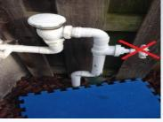
Non-testable Atmospheric Vacuum Breaker (AVB) for use on lawn sprinkler systems not under continuous pressure (note the shut off valve not permitted on sprinkler side (downstream) of the device
