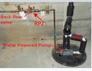
Water assisted backup sump pump protection with a required RPZ backflow prevention assembly
