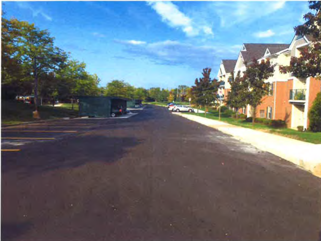
New parking lot asphalt, car port concrete, and replaced concrete sidewalk
