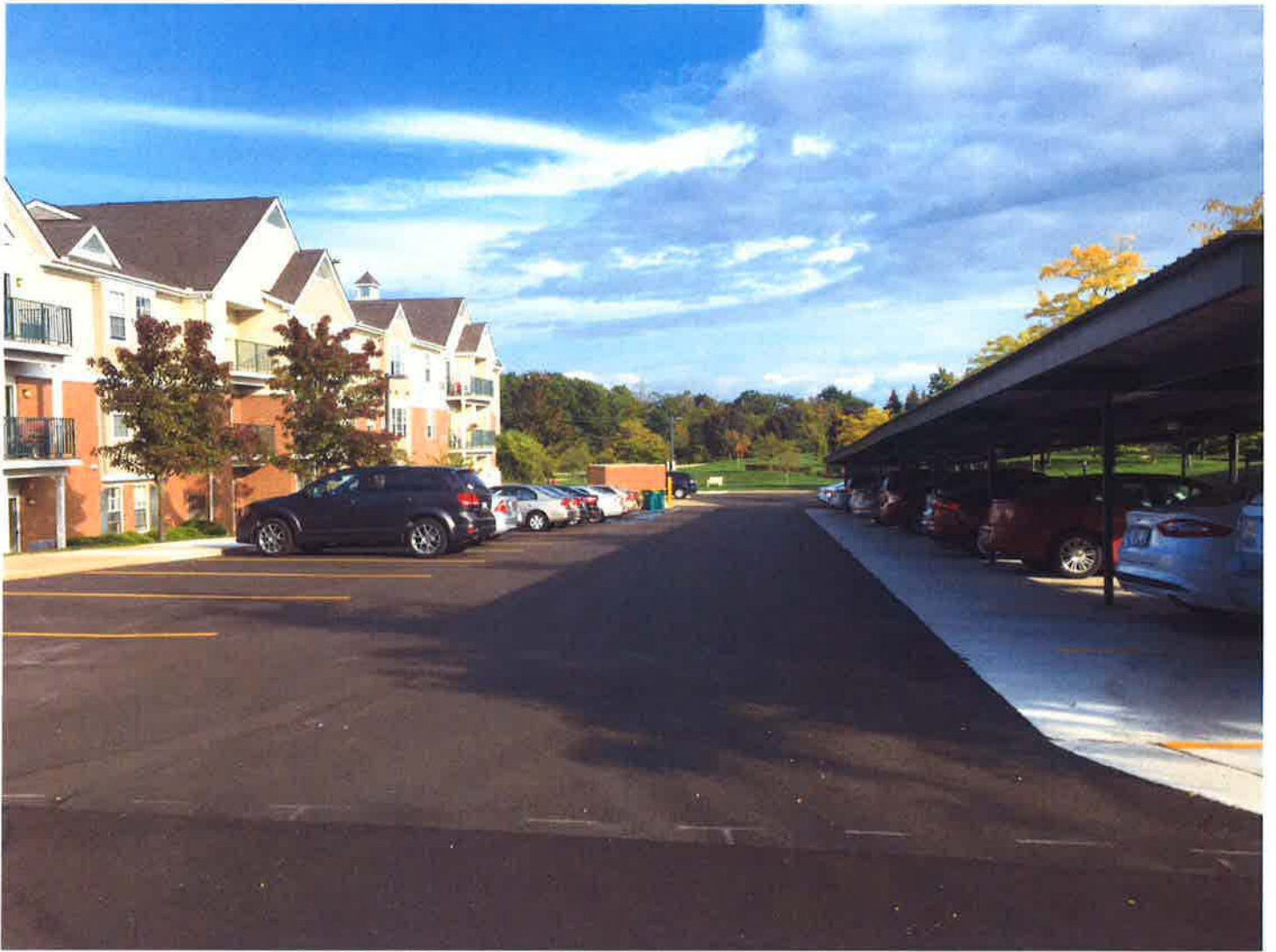
New asphalt, curb, concrete car port pads at the rear of the main building.
