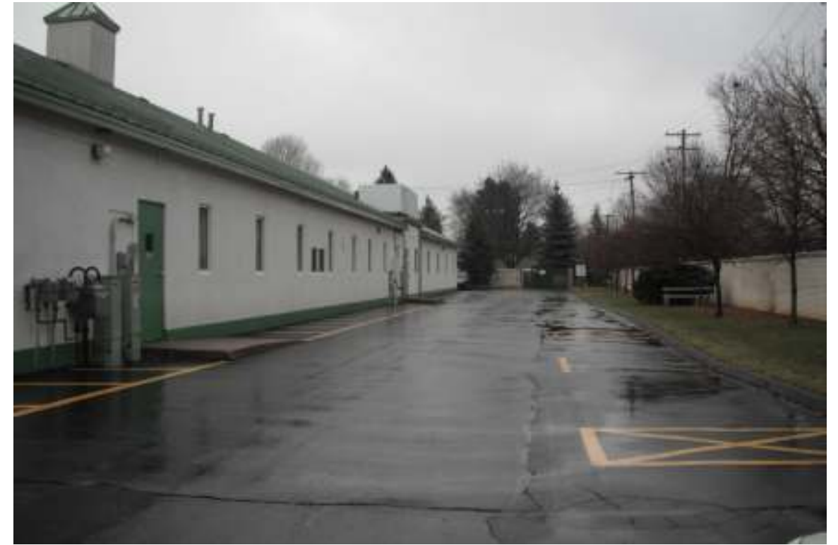
18. Commercial center rear – Southeast quadrant
