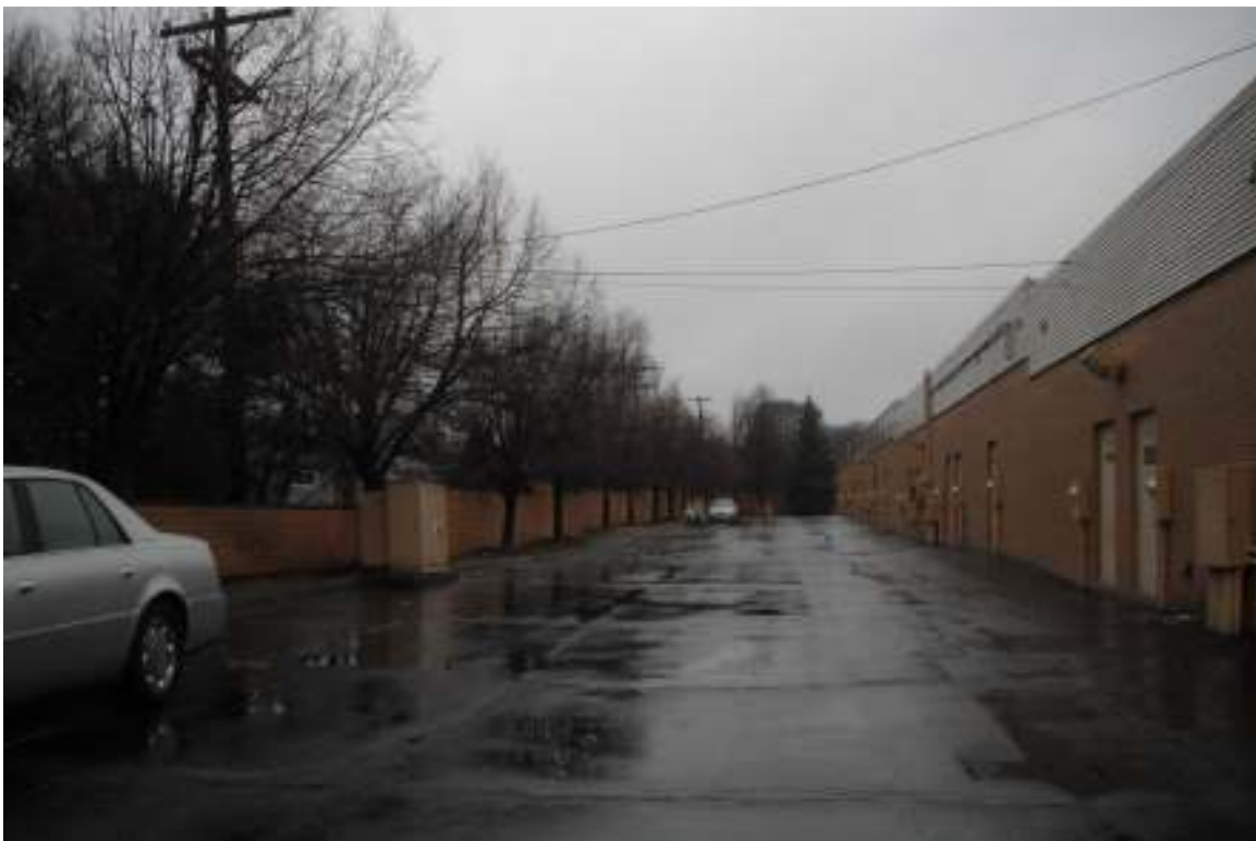
19. Commercial center rear – Southwest quadrant
