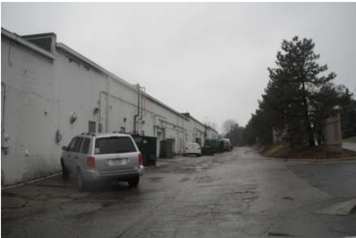
3. Rear of commercial center – Unenclosed vehicles and dumpsters
