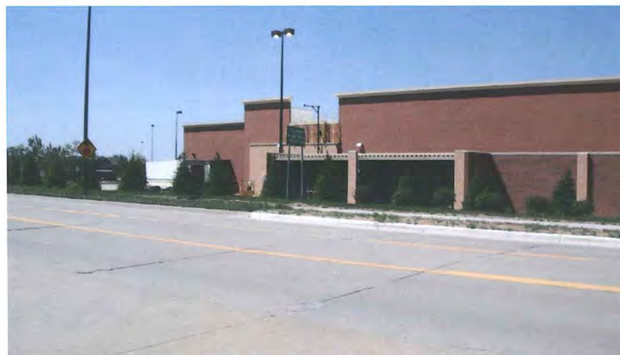
Looking southwesterly from the east side of Town Center Drive
