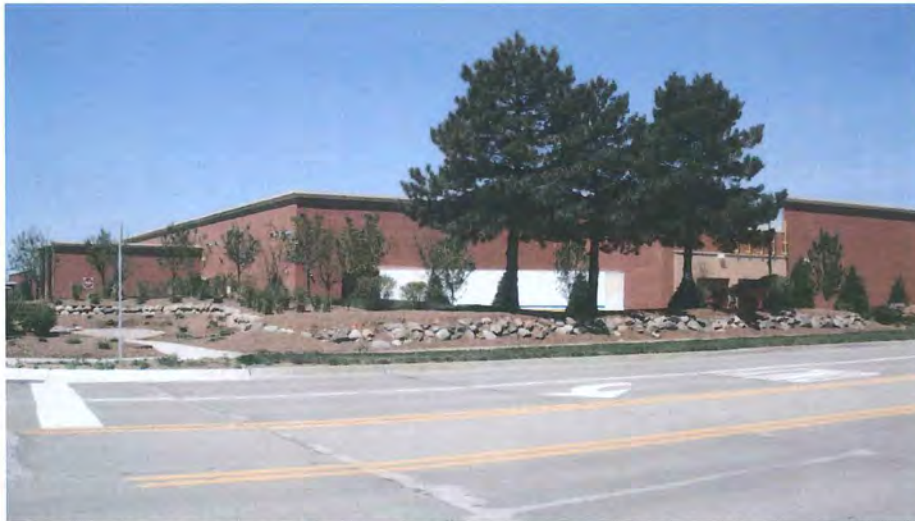
Looking west from the intersection of Town Center Drive and Eleven Mile Road
