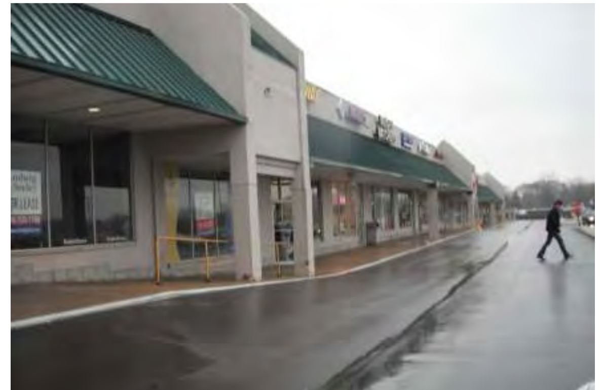
4. Front of commercial center
