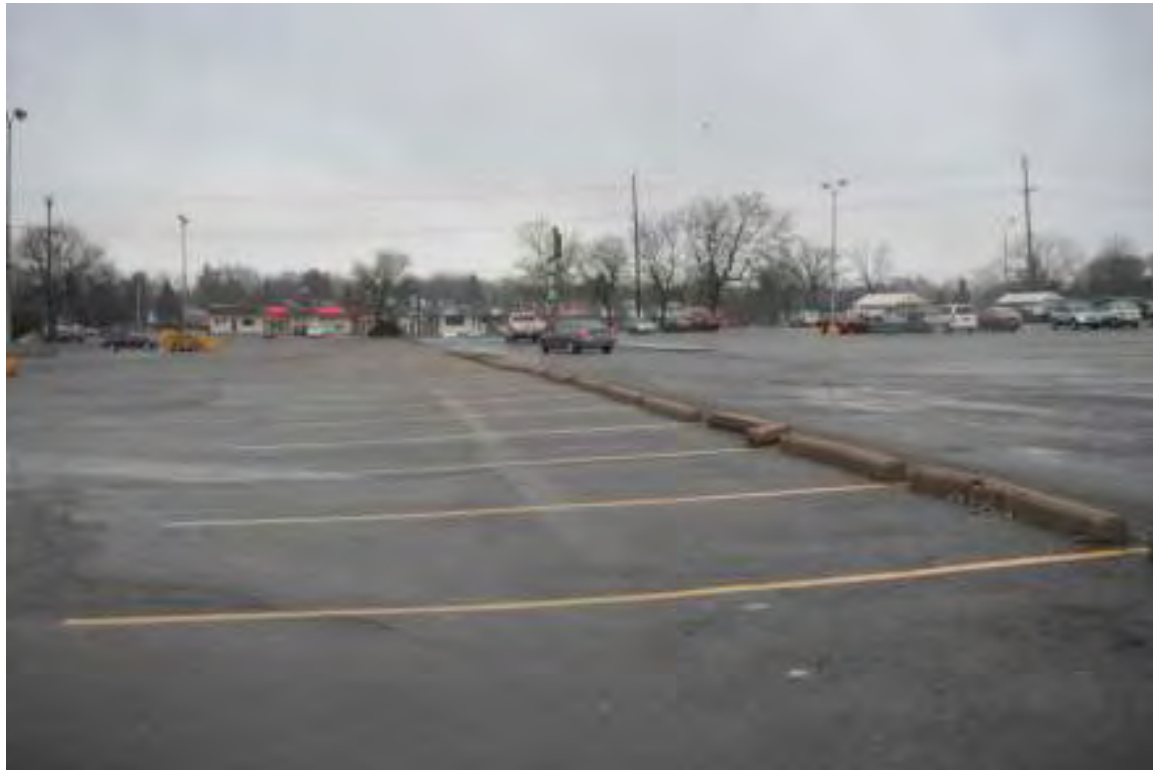
5. Parking lot – Central bumper blocks
