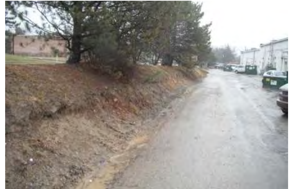
2. Rear of commercial center – Berm erosion; exposed meters, pipes, and Conduit; and unenclosed dumpsters
