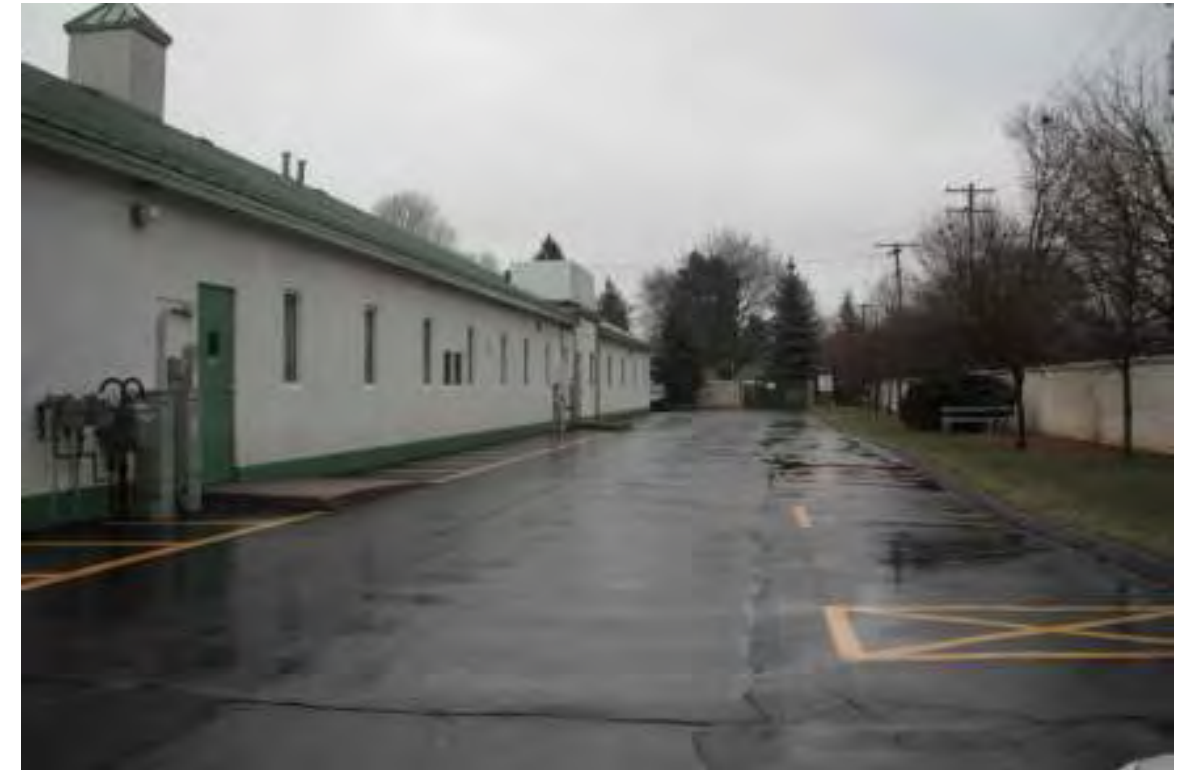
18. Commercial center rear – Southeast quadrant
