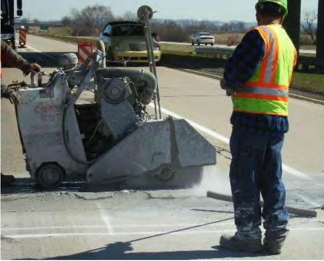
Saw Cutting Section For Removal
