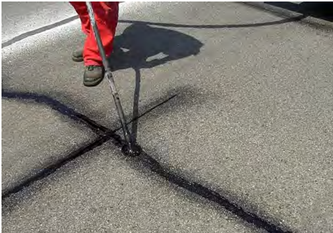
Overband Crack Seal Application
