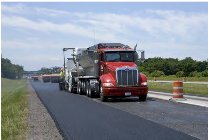
Overlay Paving Operation
