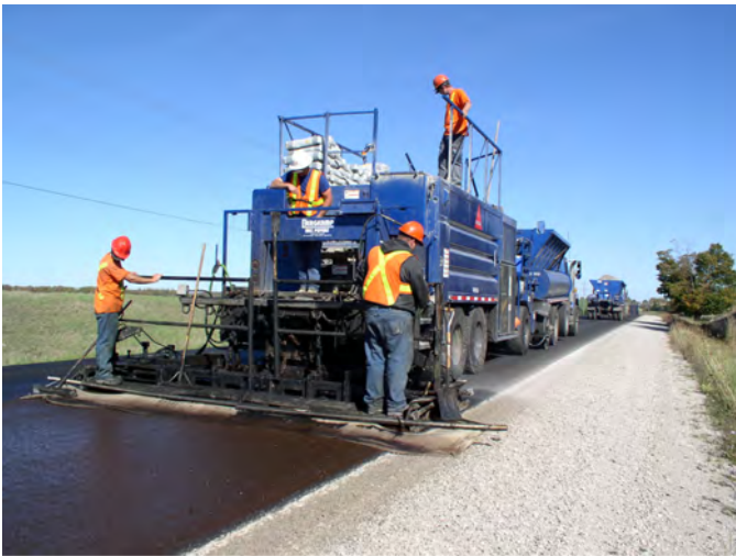
Slurry Seal Application
