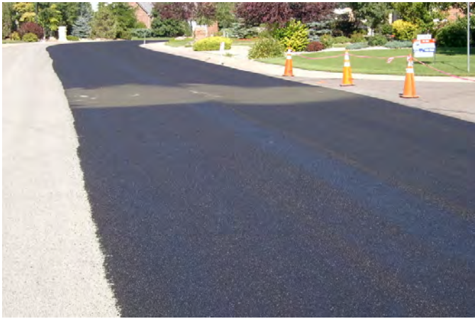
Cape Seal Application
