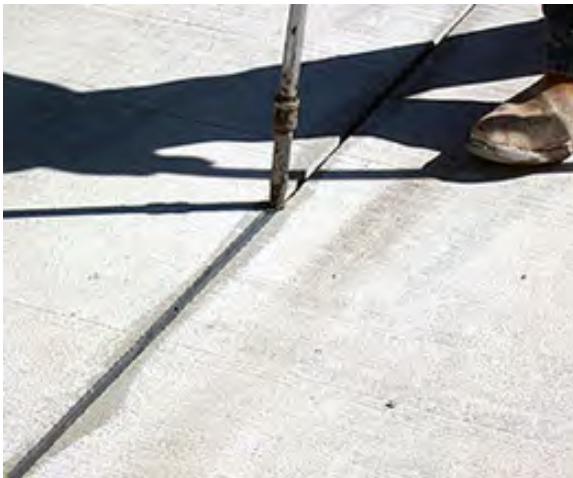
Joint Sealant Being Applied
