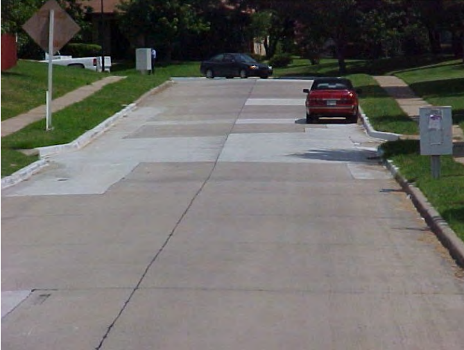
Subdivision Street After Patching And Slab Repair.
