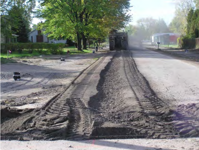
Pulverizing Existing Pavement Prior To Overlay
