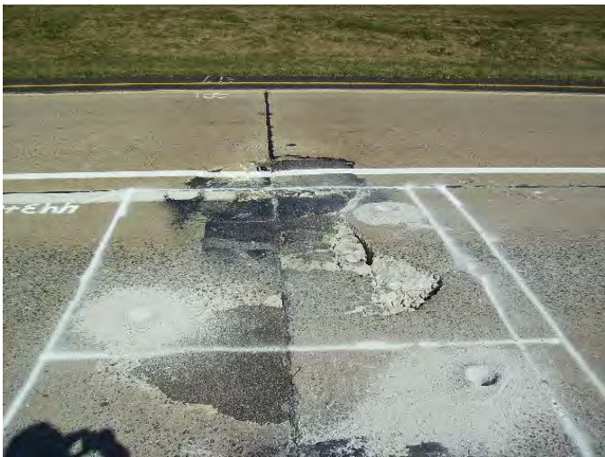
Failed Section Marked For Replacement
