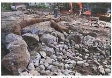
methods to alleviate a downstream erosion problem. High storm sewer outlet velocities were found to be the cause of stream bank erosion problems within the Nichols Arboretum (nature preserve).
