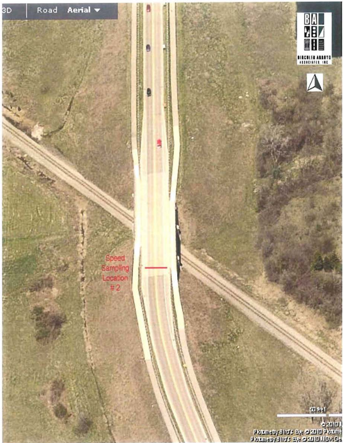
Figure 6. West Park Drive, Second Section South from West Road
