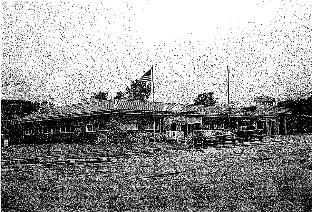
Fire Station Re-roof and interior renovation
