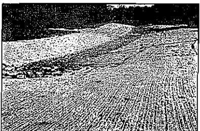
Mulch blankets used to reduce soil erosion and stabilize new plant material
