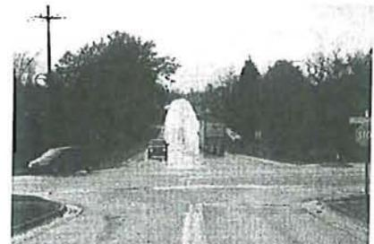
Misaligned lane configurations may require guideline striping through intersection.
