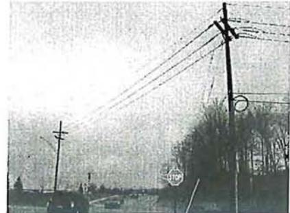
Box span signals may help to avoid conflicts with diagonal DTE Energy overhead wires.
