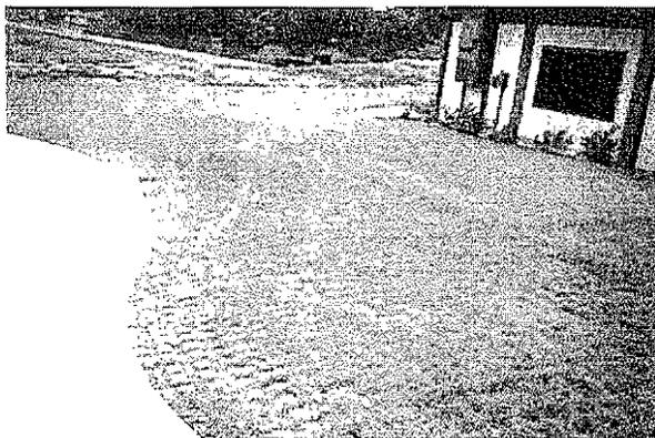
Turf pavers used for an emergency access drive
