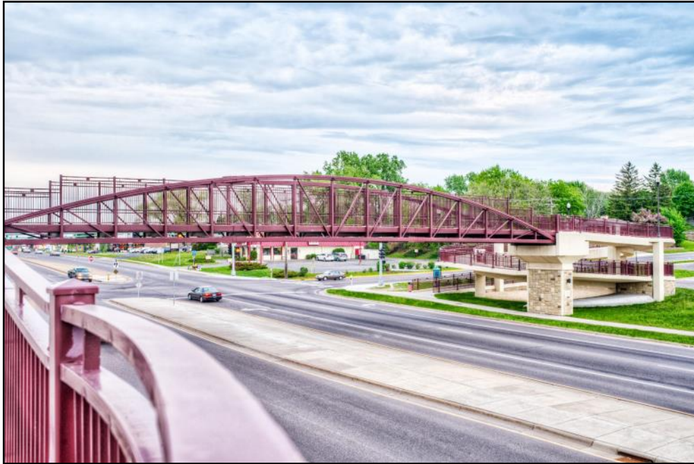
Figure C10: Pedestrian bridge with accessible switchback ramps in Columbia Heights, Minnesota. Photo courtesy of C.S. McCrossan
