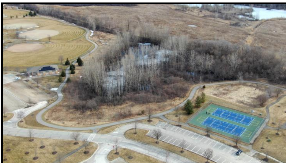
Figure B9: the ITC Trail is a prime example of non-motorized infrastructure in the City of Novi
