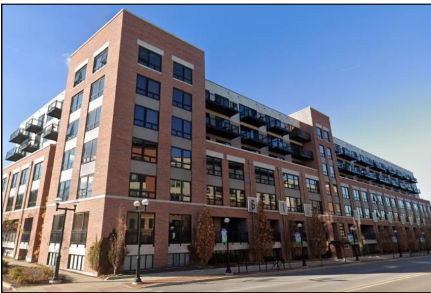
Figure D24: 618 South Main Apartments in Ann Arbor provide structured parking within the building, high quality building materials, offsets in the architecture, and balconies for its residents
