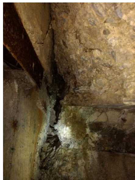
Figure 2: Bishop Ck Culvert WB travel edge
