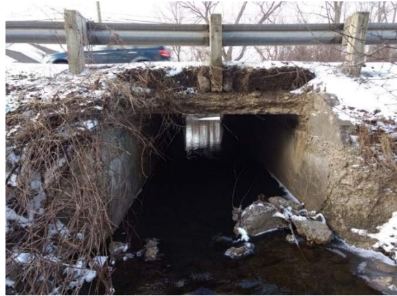
Figure 10: Ingersol Ck Culvert, south side
