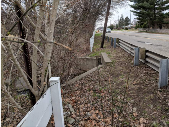
Figure 3: Bishop Ck Culvert, south side looking west
