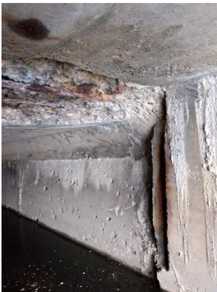
Figure 1: Bishop Ck Culvert south curb line
