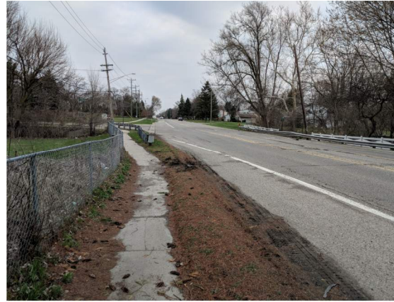
Figure 4: Bishop Ck Culvert, north side looking east
