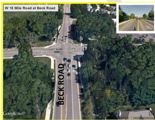
Figure 21. Beck Road at 10 Mile Road
