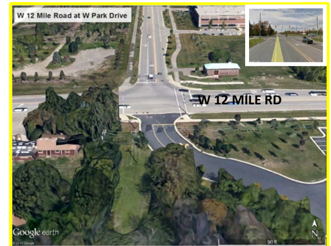
Figure 25. W Park Drive at 12 Mile Road
