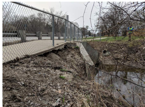
Figure 8: Ingersol Ck Culvert, north side looking west
