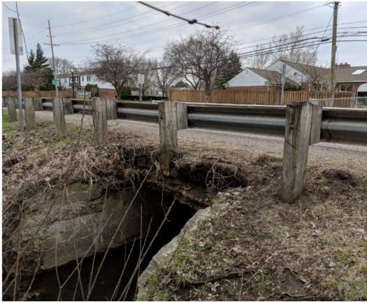
Figure 9: Ingersol Ck Culvert, south side
