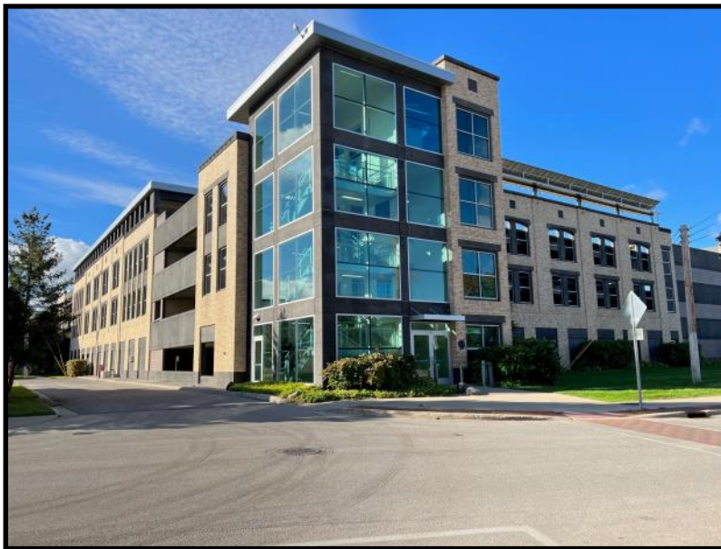
Figure E27: Parking structure in Traverse City
