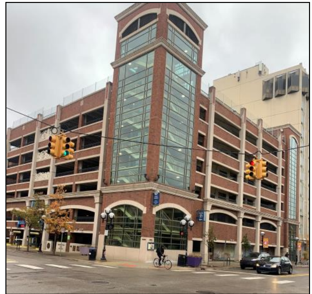
Figure E26: Parking structure with screening and high quality material in Ann Arbor
