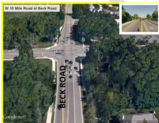
Figure 21. Beck Road at 10 Mile Road
