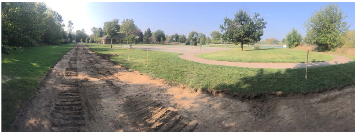
Segment # 4064: Regional pathway connecting the ITC trail at ITC Community sports park to Eight Mile road, currently under construction
