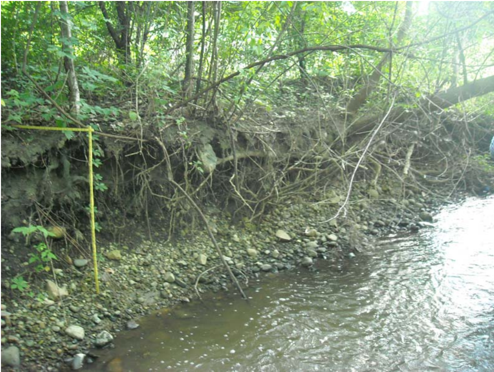
Undercutting Bank, looking downstream
